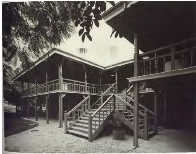
Examples of modern balconies and balustrading.
