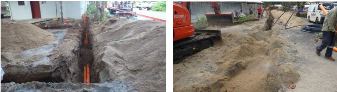
(Above) New Power Conduit being run between the two Toilet Blocks
