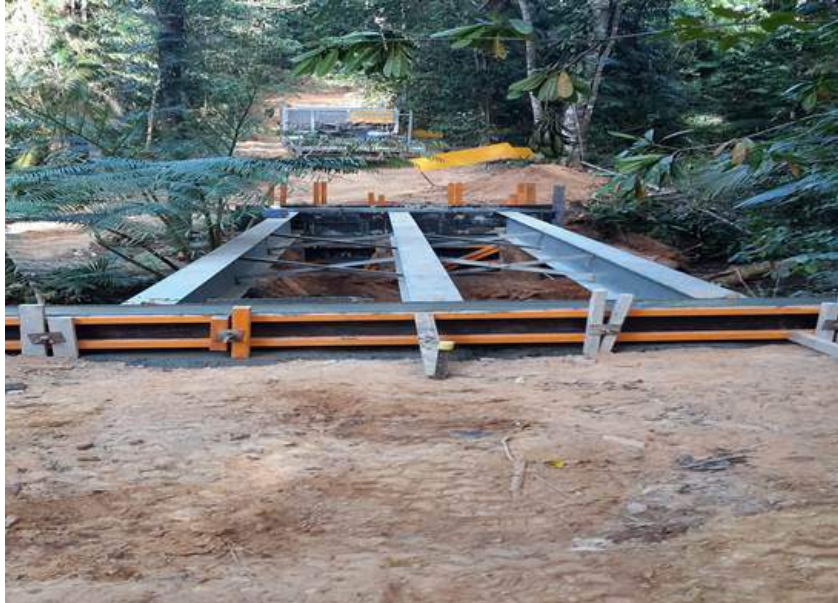
(Above) China Camp Fischer's Bridge (first Log Bridge)
