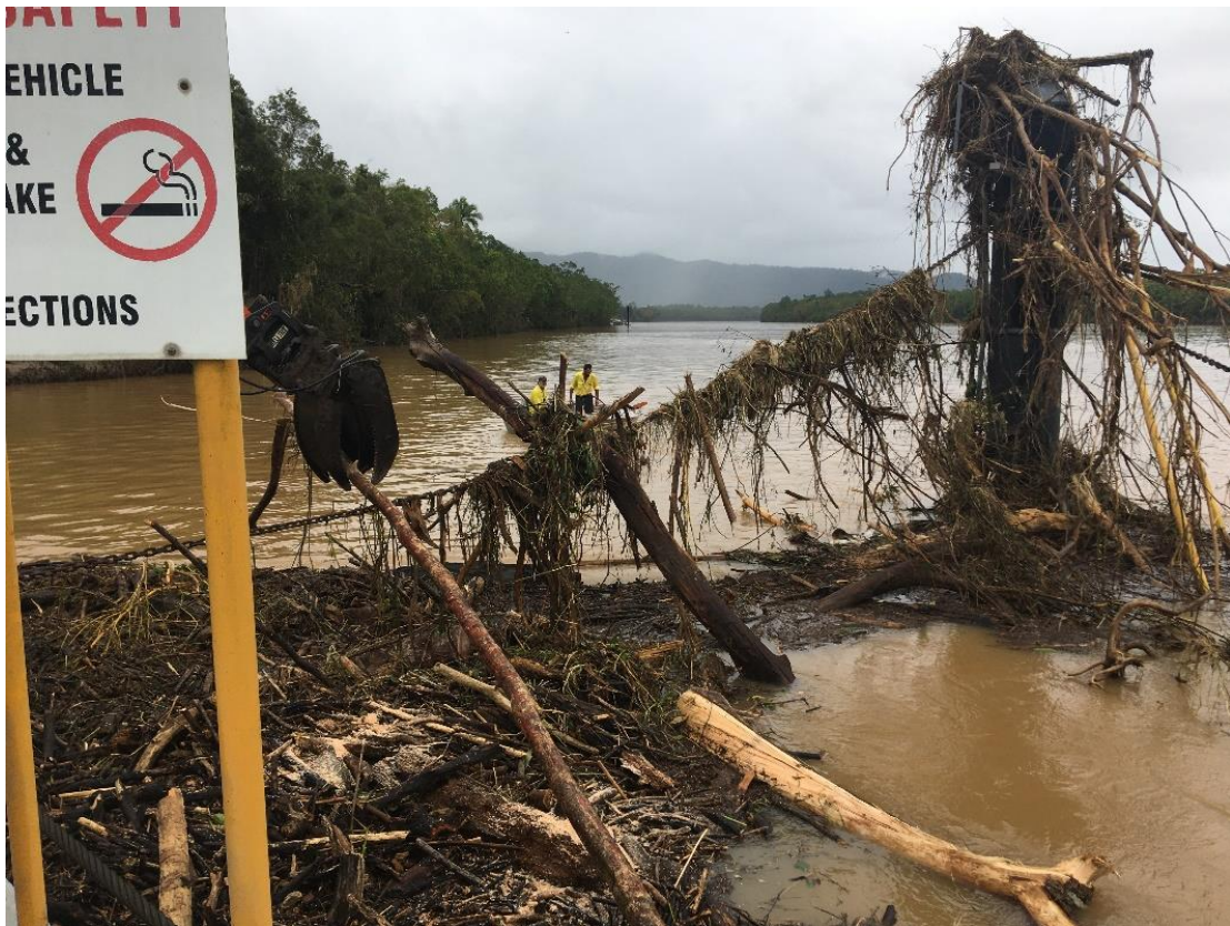
Image: Crew clearing debris to unchain Daintree Ferry
