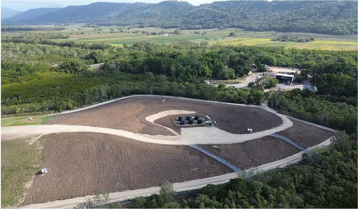
Image: Final landfill capping completed, Killaloe
