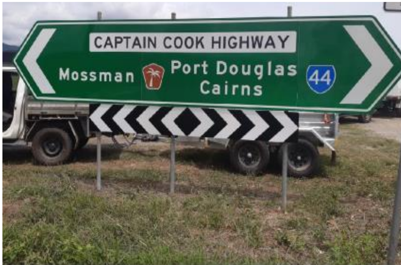
Image: New directional signage installed at Captain Cook Highway
