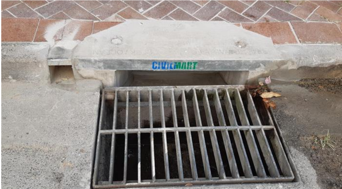
Image: Reconstructed stormwater pit on Front Street
