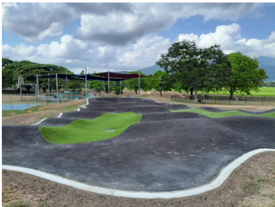
Image: Pump Track in Mossman
