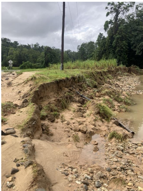
Images: Water network breaks after tropical cyclone Jasper
