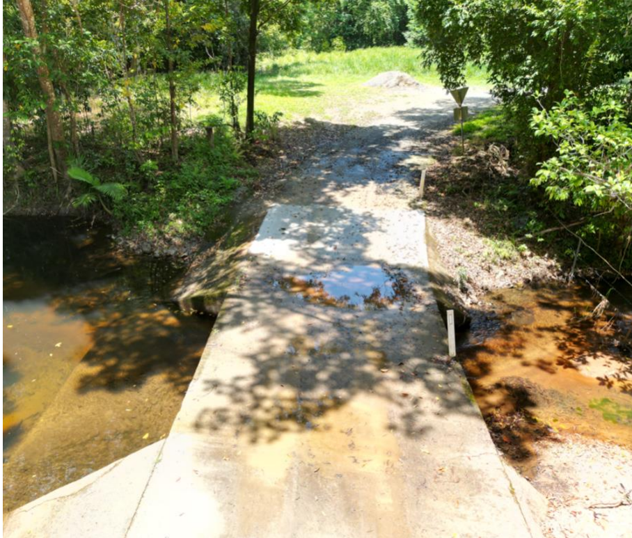
Image: Repairs to the Crystalbrook Road Causeway
