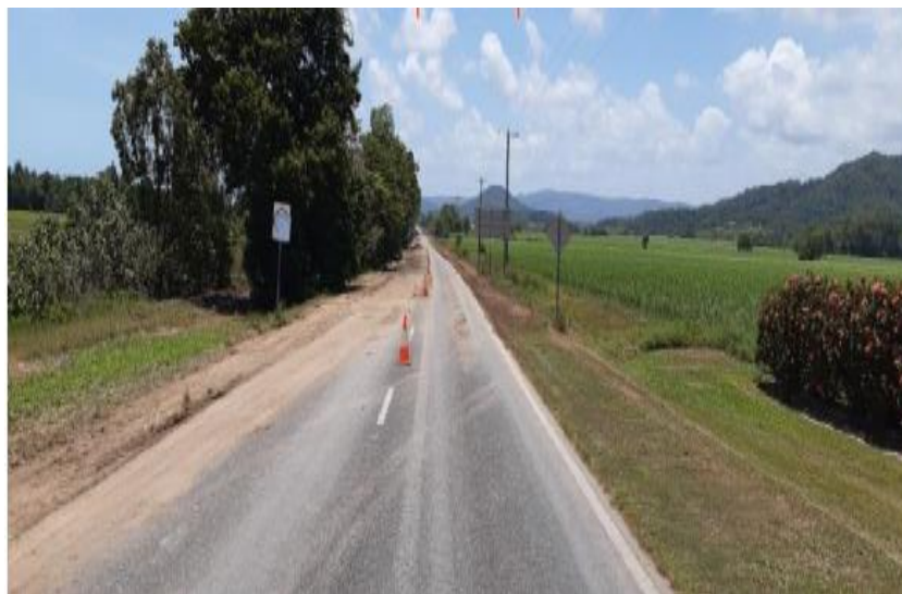
Image: Post-grading along Mossman-Daintree Road
