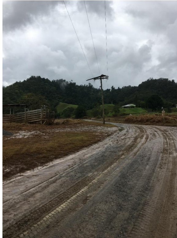
Image: Flood debris on power pole Upper Daintree
