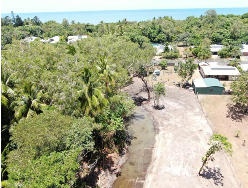
Image: Drain clearing at Marlin Drive, Wonga Beach
