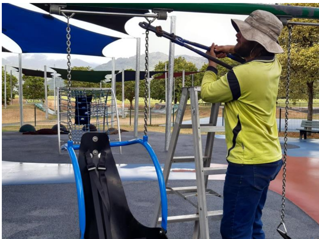
Image: Playground maintenance / swing replacement
