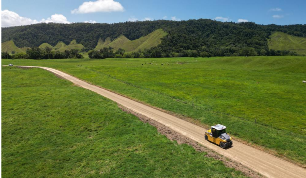
Image: Grading renewal along Douglas Creek Road
