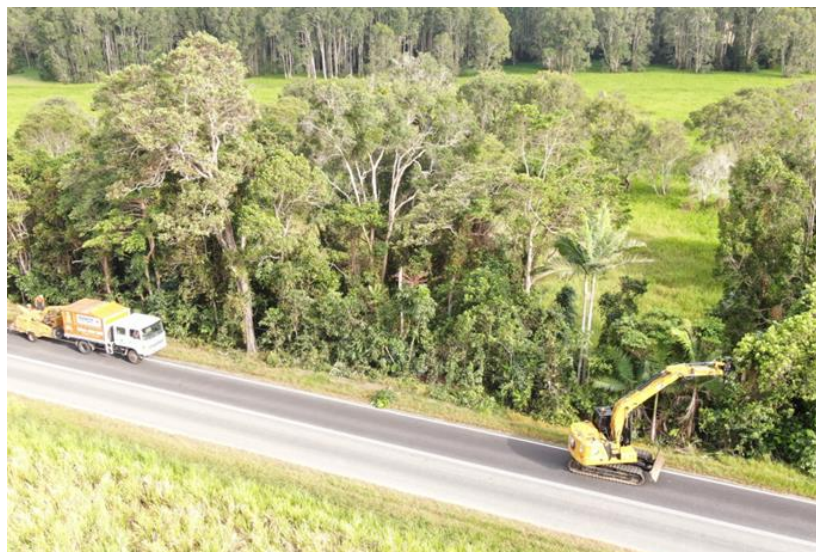
Image: Roadside vegetation trimming and removal
