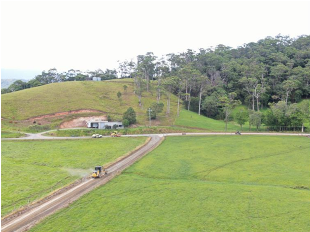
Image: Grading along Mary Lane
