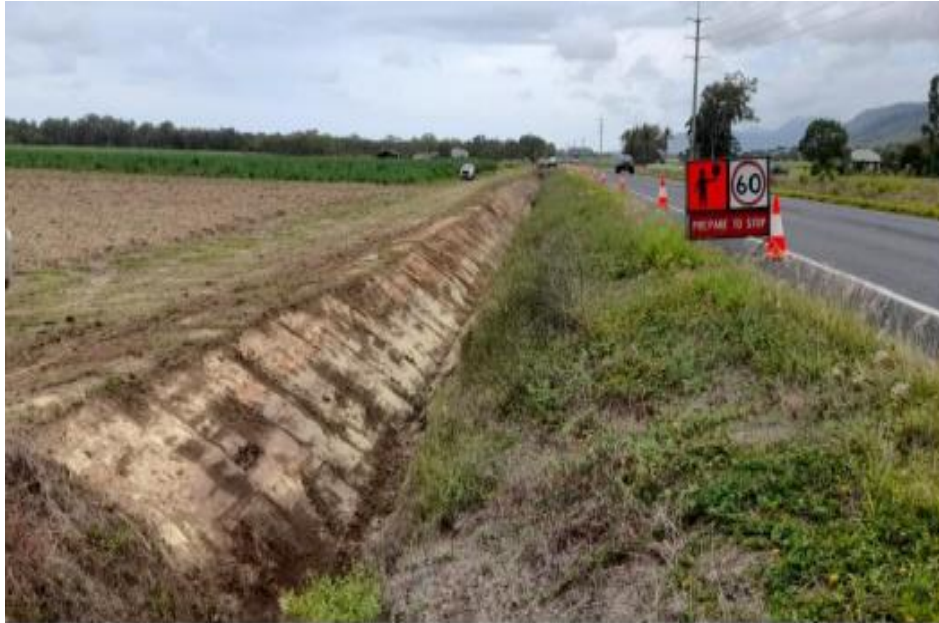
Image: Drain clearing along Captain Cook Highway in November
