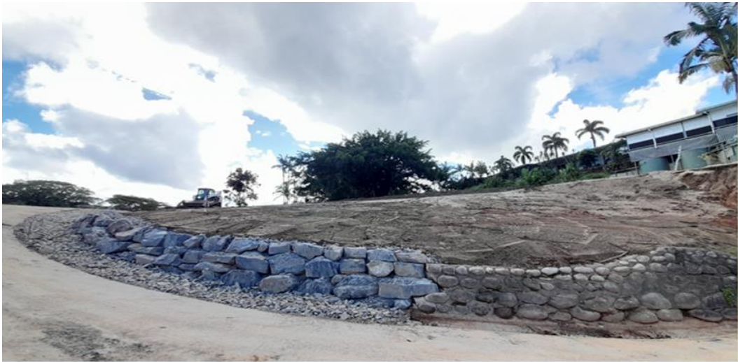
Image: Daintree boat ramp slopes in preparation for hydro mulching
