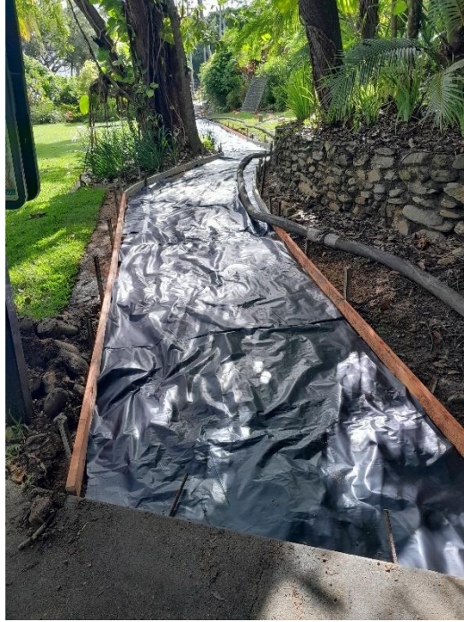
Image: Works in Progress Little Cove Upgrade
