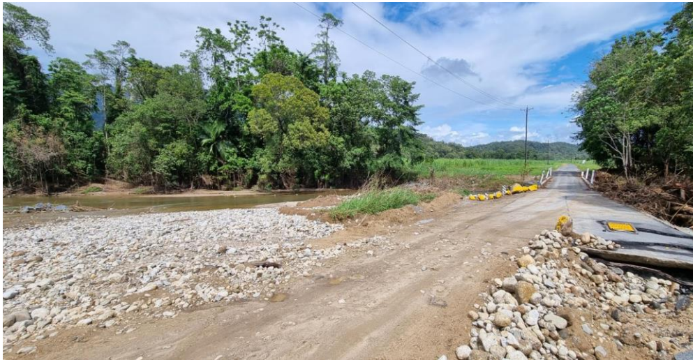
Image: Before the repairs to Pollocks Bridge
