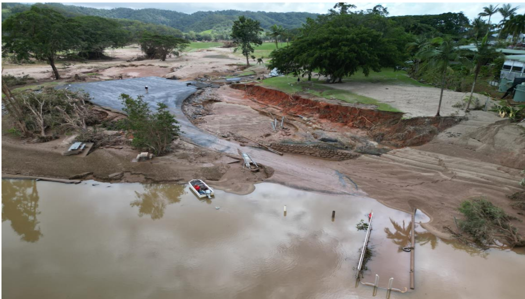
Images: Post flood damage to the Daintree Village boat ramp car park Ordinary Council Meeting - 30 April 2024
