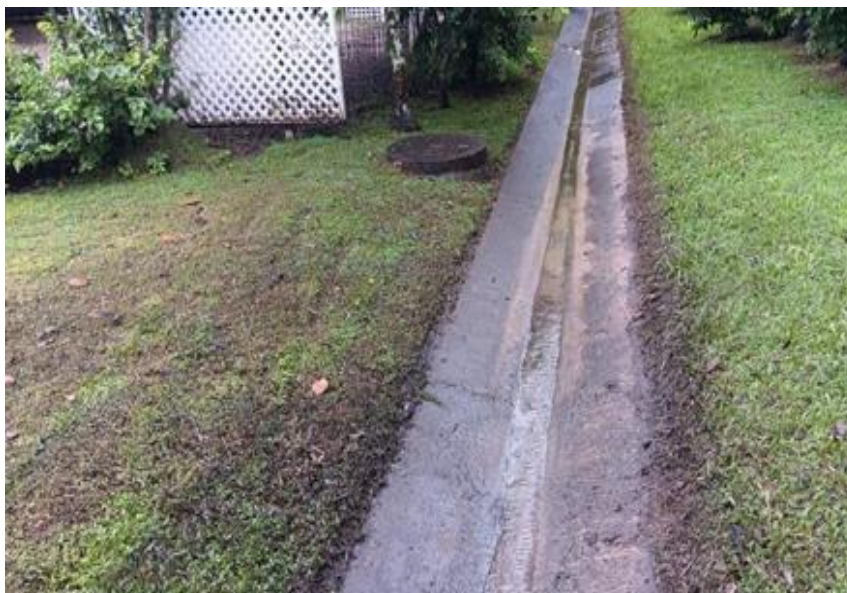
Image: Drain cleaning - Mowbray Street
