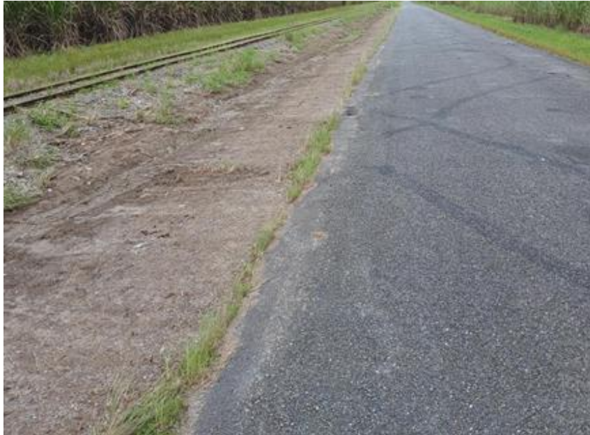
Image: Drain clearing – Syndicate Road
