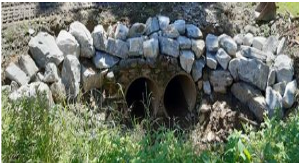
Image: Drain repairs - Upper Cassowary Road Ordinary Council Meeting - 30 April 2024
