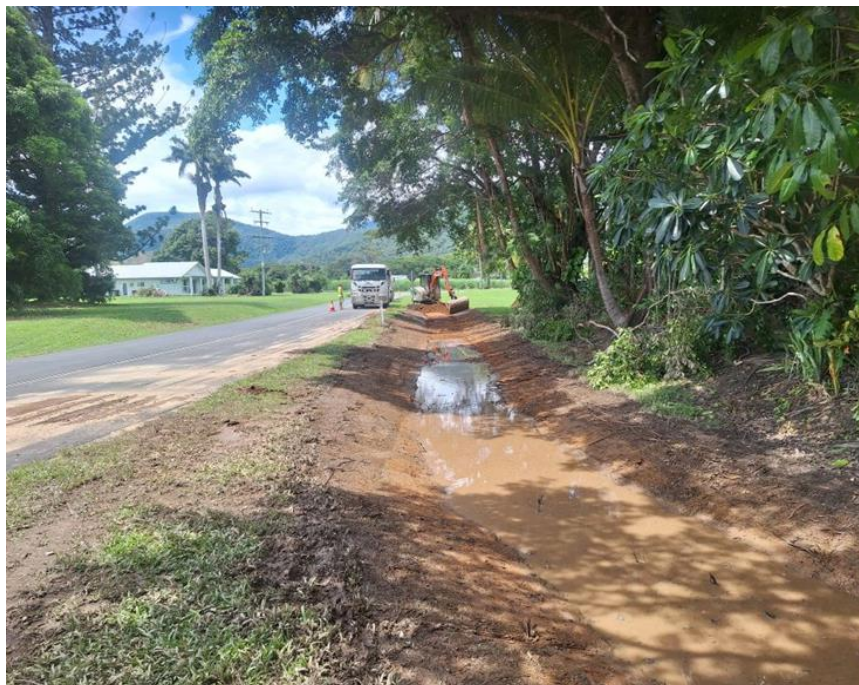
Image: Drain clearing - Mowbray River Road
