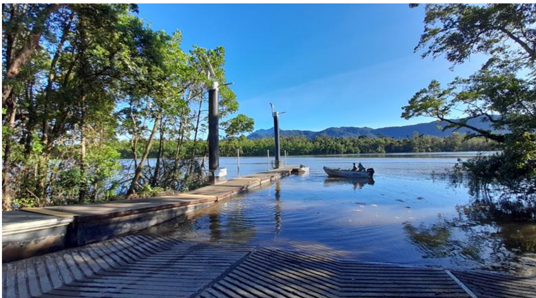
Image: Road-TEK repairs complete – Lower Daintree boat ramp
