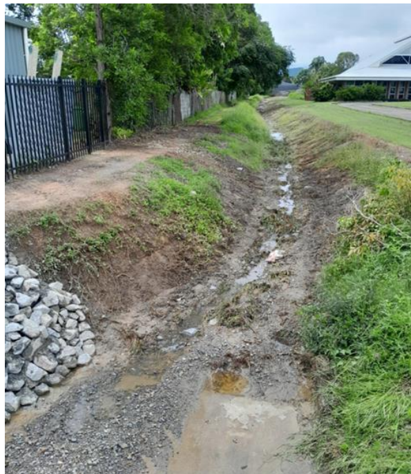
Image: Drain cleared – Port Douglas
