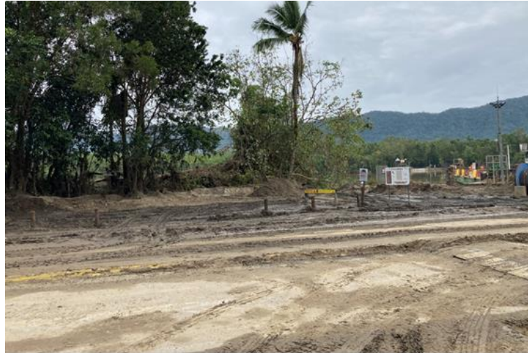
Image: Day 2 of Clean Up at Ferry Southern Approach
