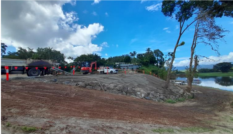
Image: Re-construction and revegetation progress
