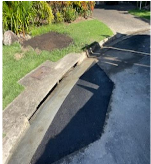
Images: Before & after entry pit repairs – Andrews Close, Port Douglas
