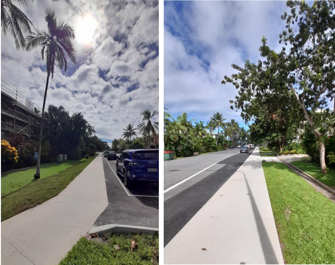
Images: Macrossan Street, East footpath renewal complete
