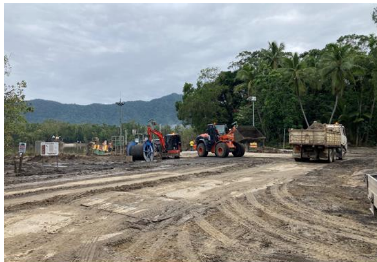
Image: Day 2 of Clean Up at Ferry Southern Approach
