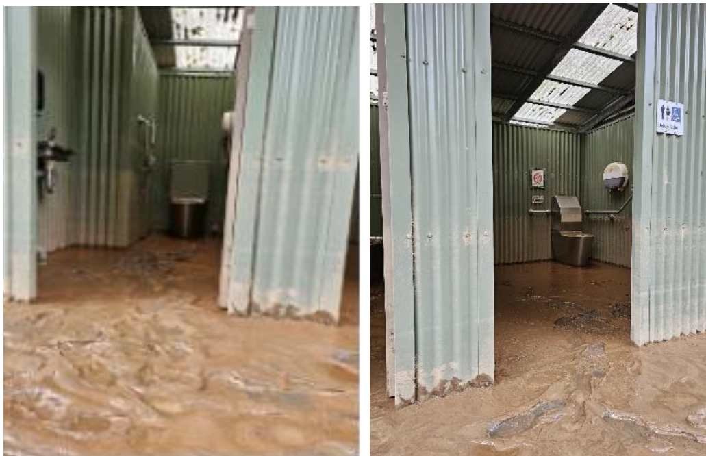
Images: Daintree Ferry Toilet Block North Side
