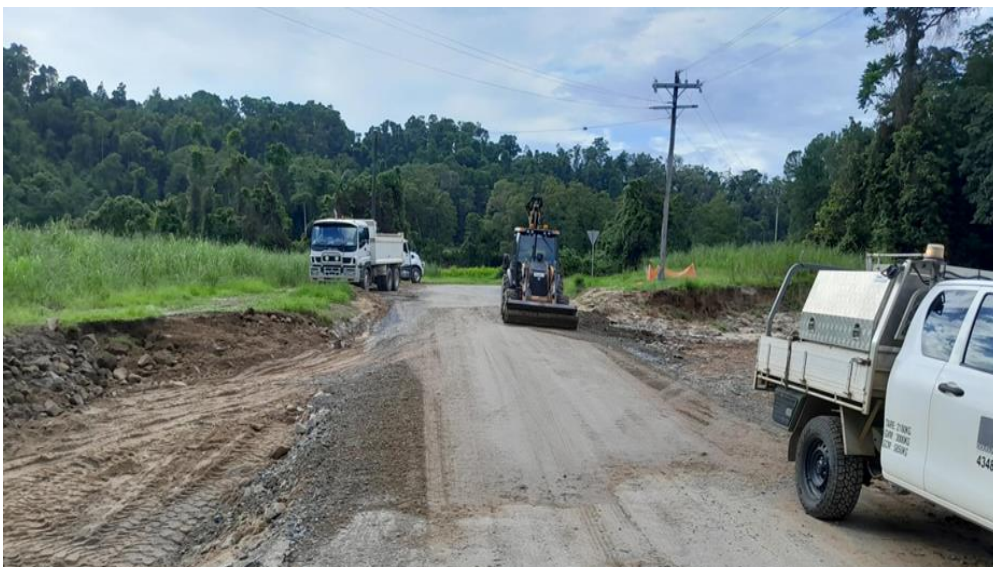
Image: Repairs to the approach of Pollocks Bridge
