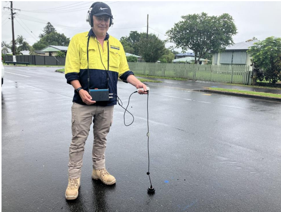
Image: Leak Detection expert
