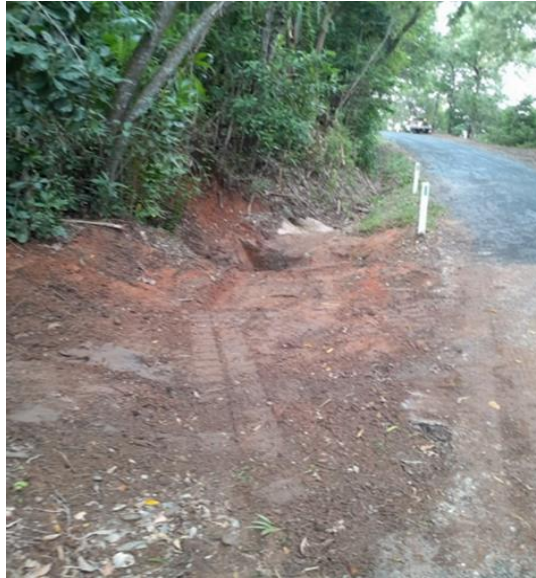
Image: Drain and road edge clearing at Island Point Road
