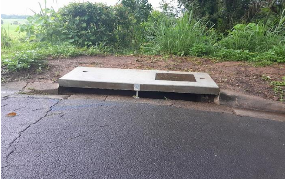
Image: Newly replaced side entry pit lid
