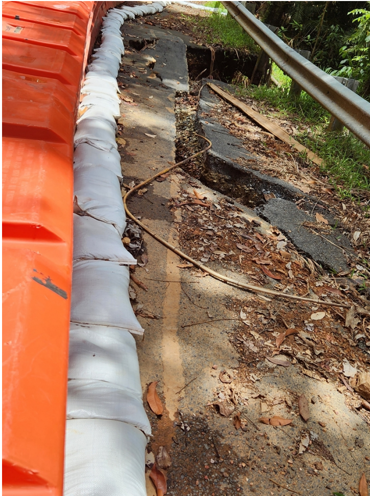
Image – Tension crack on Cape Tribulation Road
