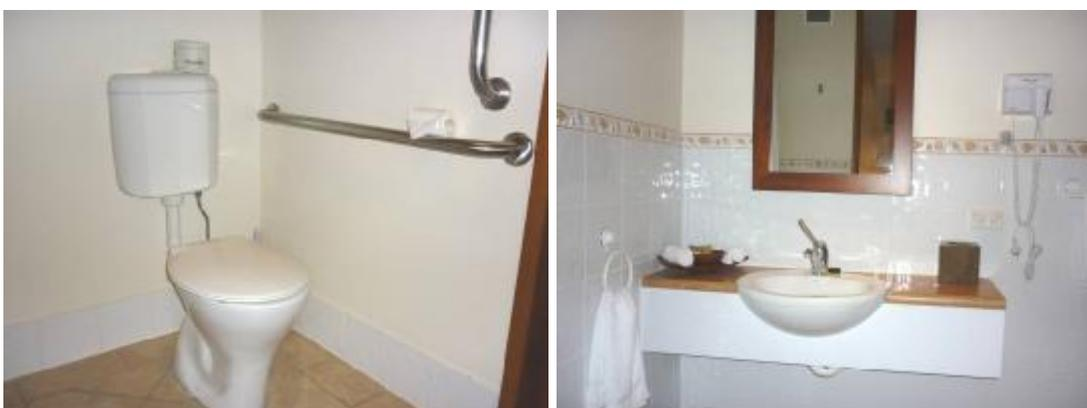
A grab rail is fitted beside the toilet and is mounted 855mm from the floor to top of grab rail.
