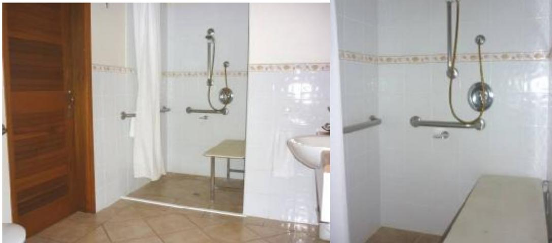
Entry into the accessible shower and toilet is through a door with a clear width of 781mm. There is also a sliding door from the bedroom.
