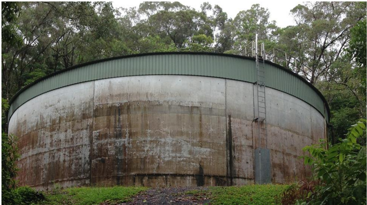
Figure 9. Whyanbeel clearwater reservoir
