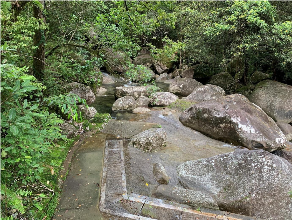
Figure 6. Rex Creek intake – race is lined with stainless steel
