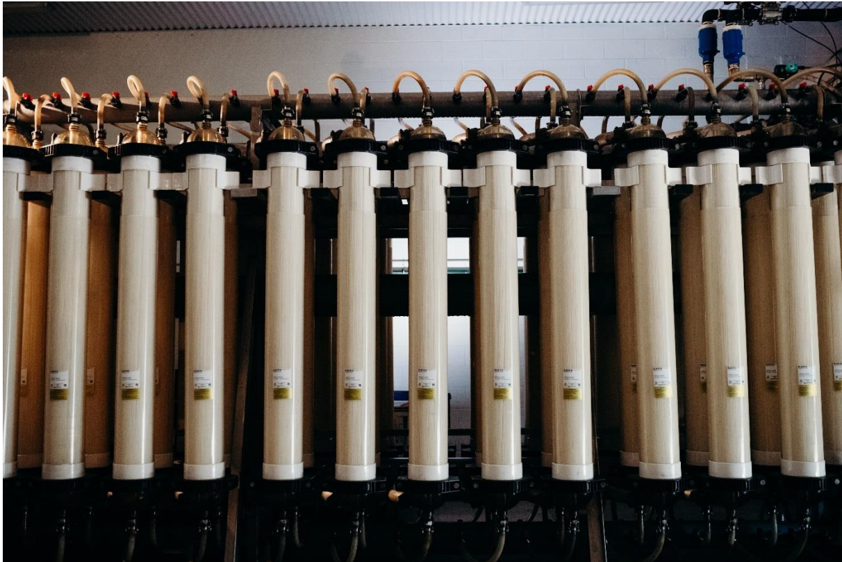
Figure 7. UF membrane rack at Mossman/Port Douglas WTP
