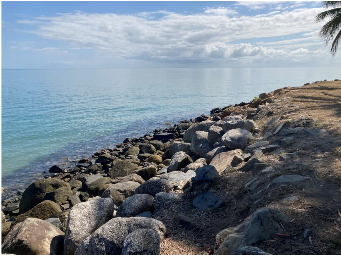
Figure 4-9: Site image from Rock wall structure at Rex Smeal Park, showing typical slope and approximate rock size distribution.
