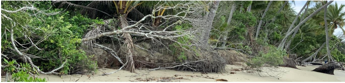
Erosion scarp on the southern end of Four Mile Beach.
