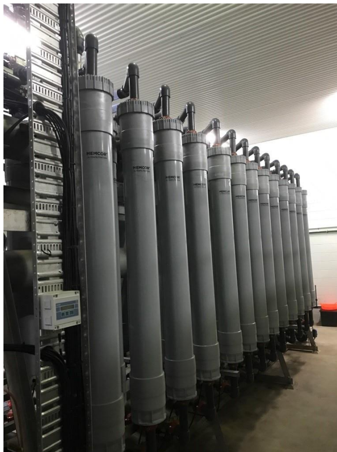
Image: Completed first membrane rack at Mossman Water Treatment Plant
