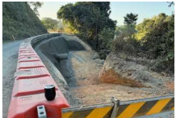
Surface covered in shotcrete.
