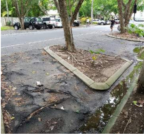
Figure 2.13: Pavement damage
