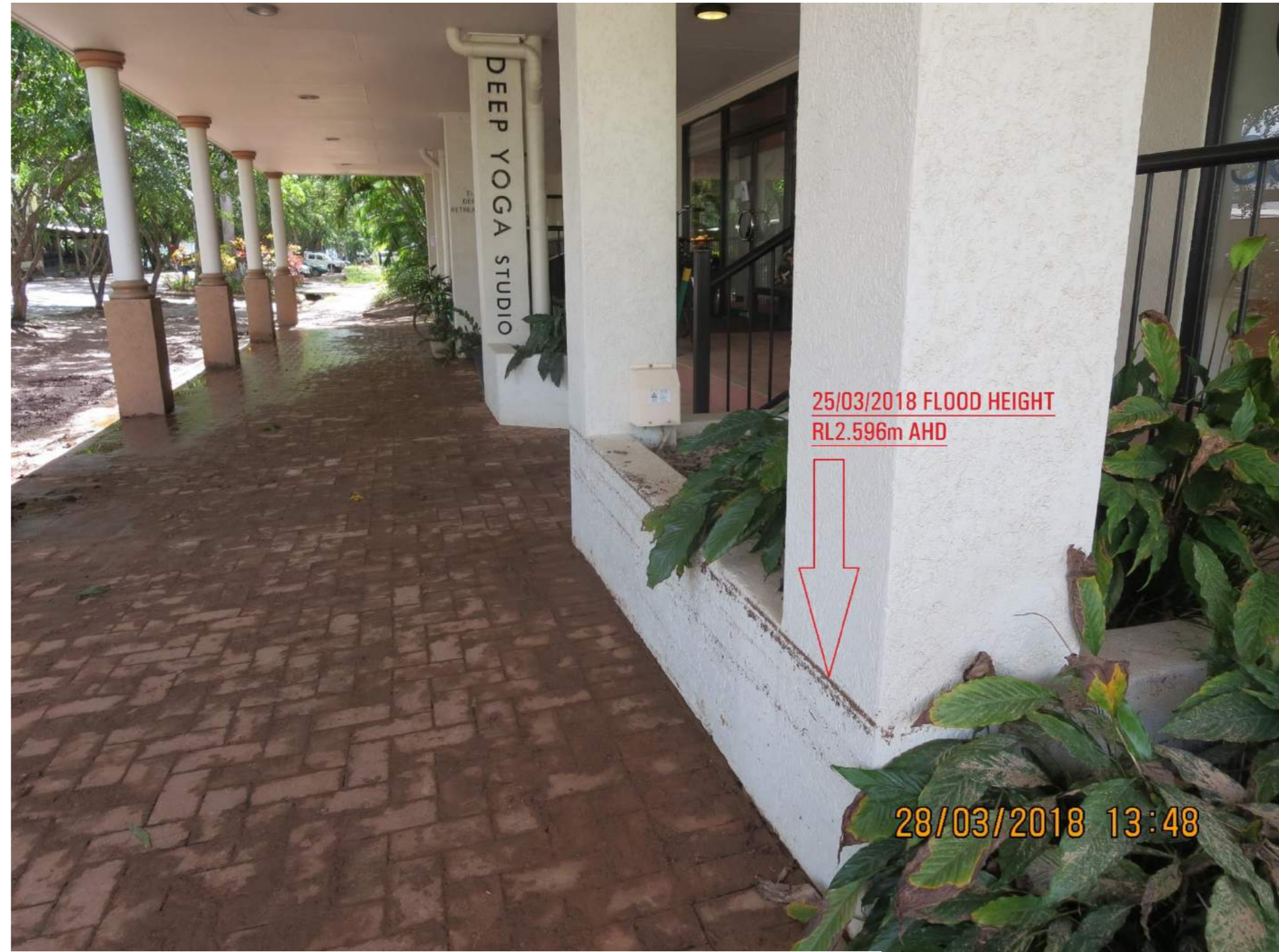
Figure 3-3: Warner Street near the corner of Grant Street flood level indicator left on building
