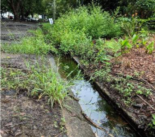
Figure 2-3: Northern kerb section
