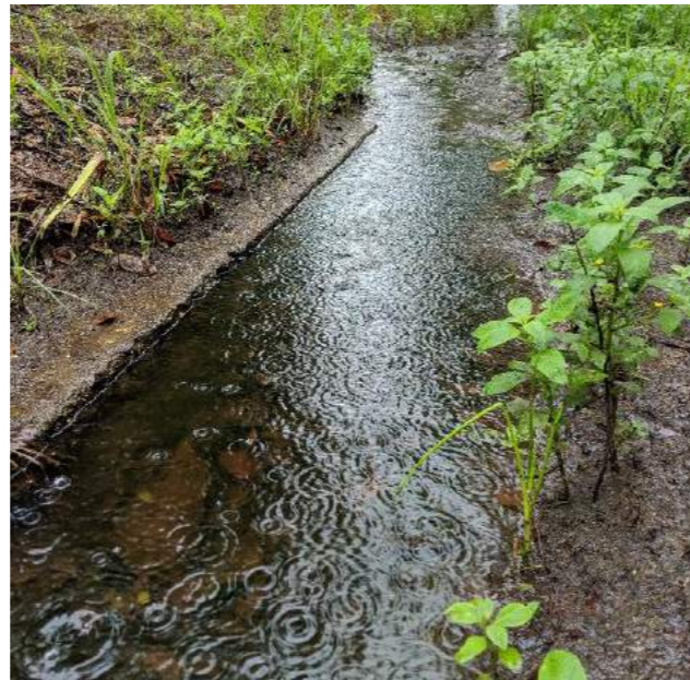
Figure 3-1: Northern side of Warner Street kerb flooding.
