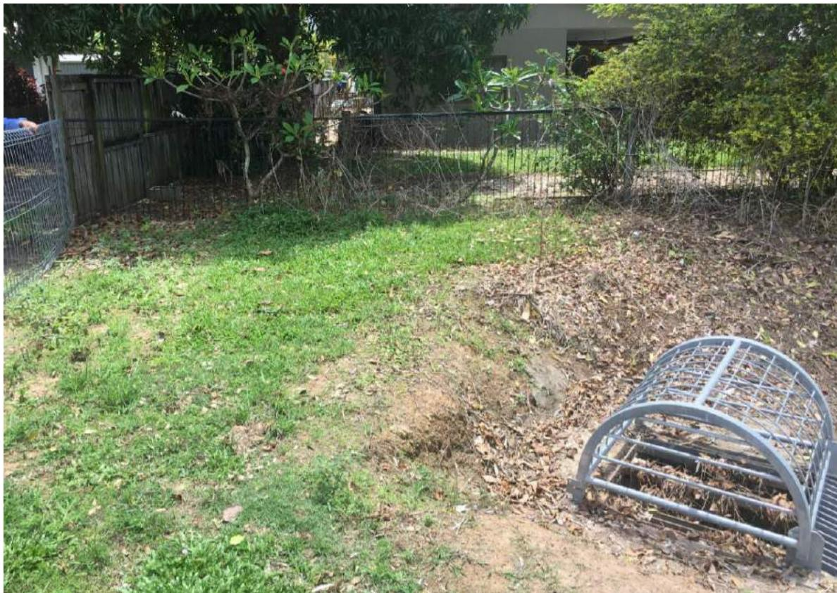
**Image 7 - Lack of freeboard between drain and adjacent lot.**
