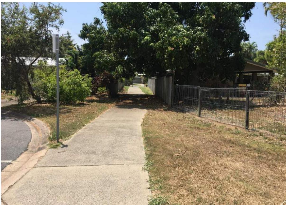
**Image 5 - Lack of definition in pathway link and overland flow path**
