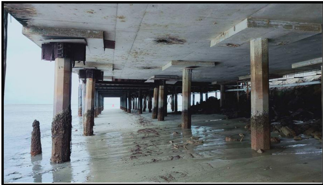
Pic 006 [piles supporting concrete jetty]
