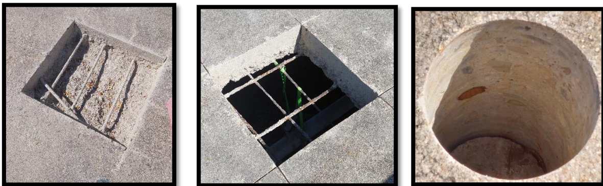
Pic 003 [one of five test holes]
