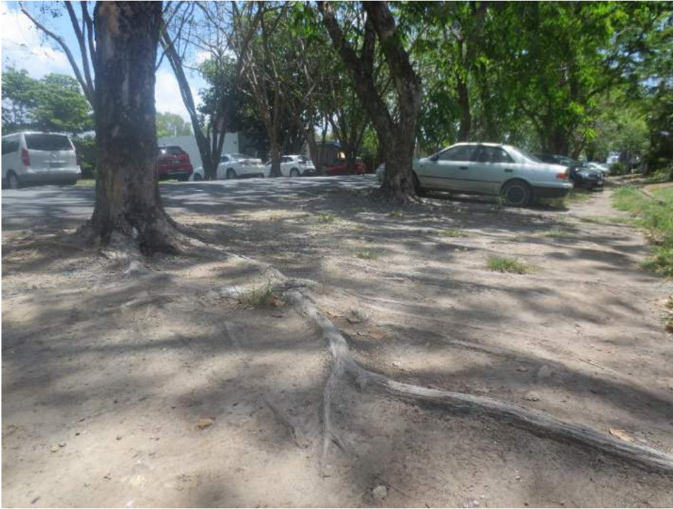
Image 3 – Typical surface roots at Warner Street
