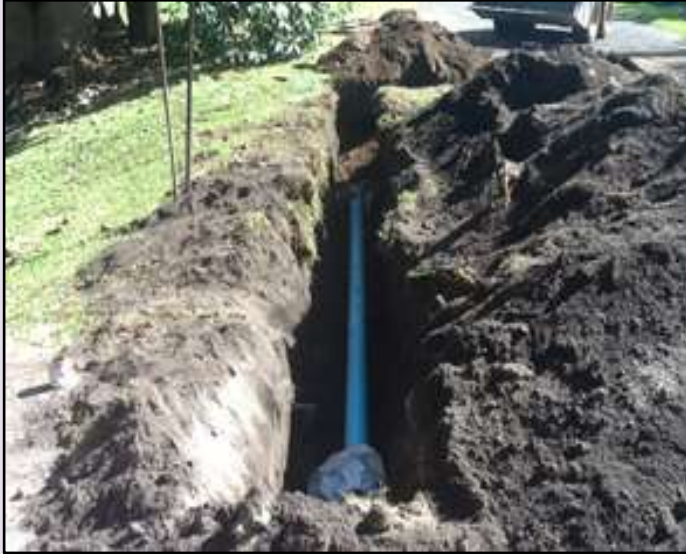
Newell Beach 100mm water main installation
