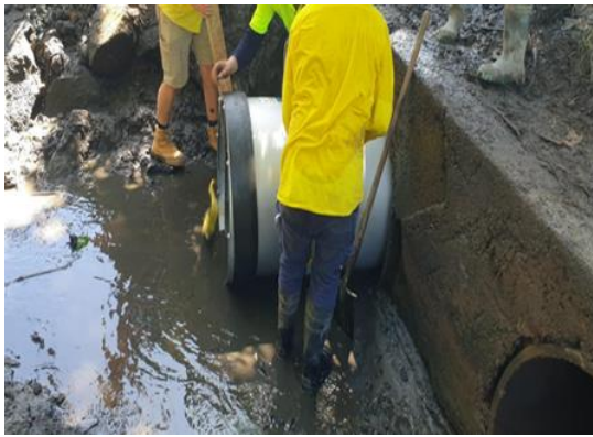
Image: Tide gate installed at Mudlo Street
