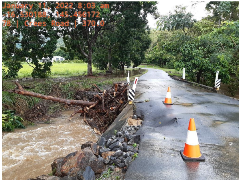
Image: Blocked drainage structure and road damage – Crees Road, Craiglie
