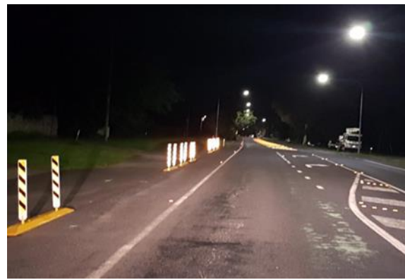
Image: Safety Kerbs and guideposts, Alchera Drive
