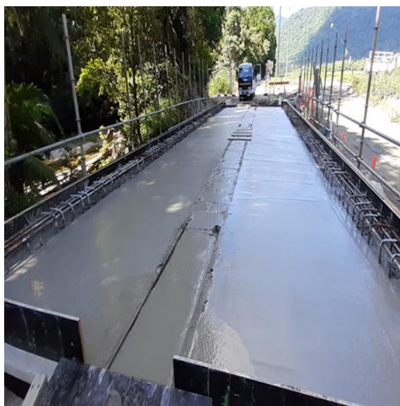
Images: Deck concrete slab pour, and stone pitching placed on the riverbank at Anich's Bridge
