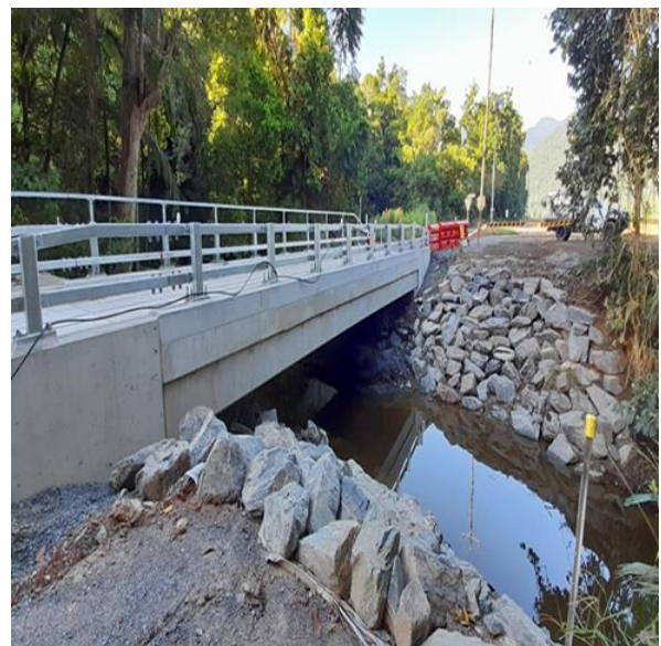
Images: Deck concrete slab pour, and stone pitching placed on the riverbank at Anich's Bridge
