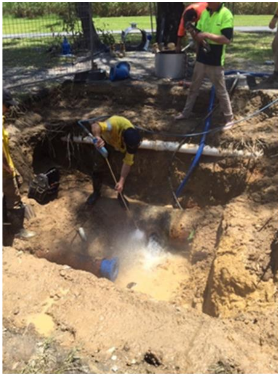
Images: Water Reticulation team replacing a faulty Wang Offtake Clamp and valve on the 450mm trunk main feeding Port Douglas reservoirs, located at the corner of Coral Sea Drive, Mossman
