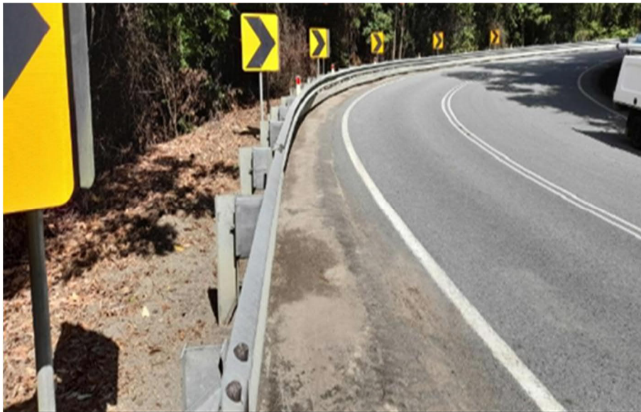
Image: Surface drainage, signs and guard rail improvements
