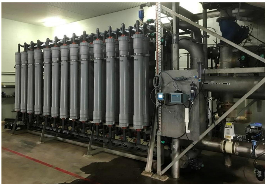
Image: New Mossman water treatment plant ultrafiltration rack
