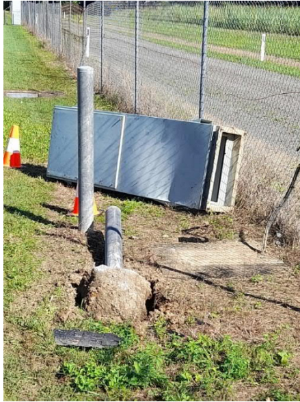
Images: Mossman Show Grounds – (Before) Car struck power outlet and after repair
