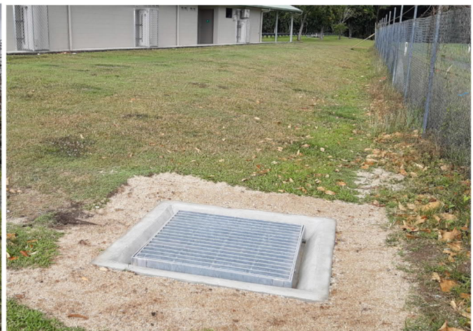
Images: Field grate installed over the drain at Coronation Park Ordinary Council Meeting - 31 October 2023
