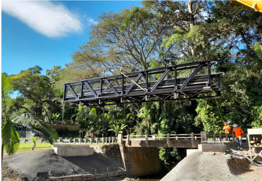
Image: New pedestrian bridge over Marrs Ck being installed
