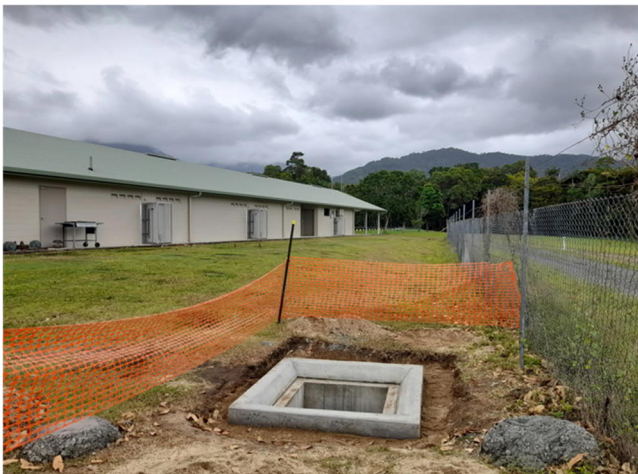
Images: Field grate installed over the drain at Coronation Park Ordinary Council Meeting - 31 October 2023
