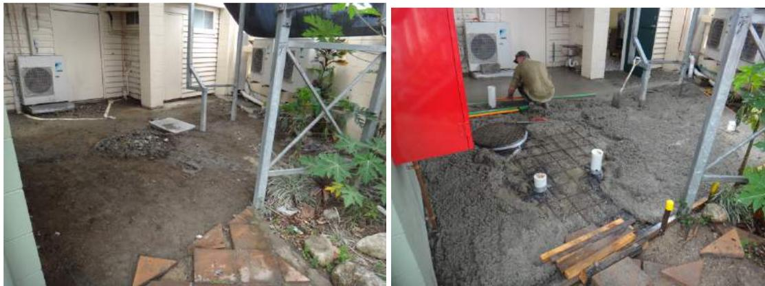
(Above) Concrete removed ready for new grease trap & new concrete being installed.
