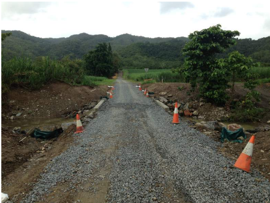
Wilkinson Rd culvert upgrade – temporary access for Christmas shutdown
