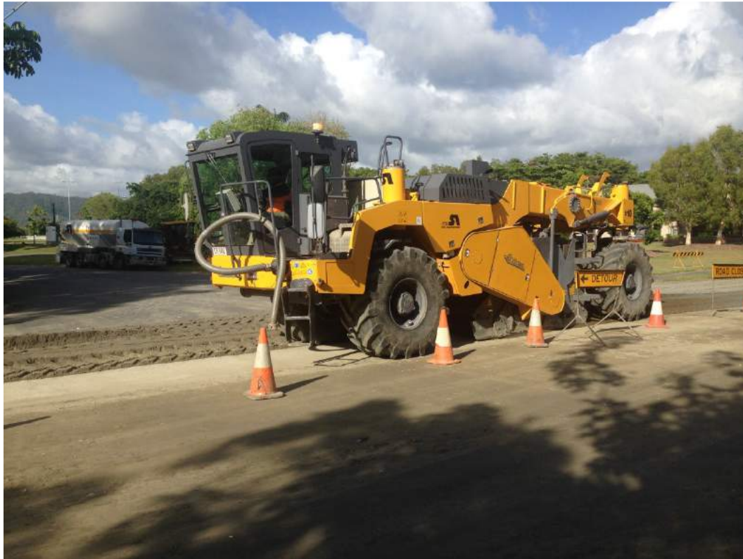
Stabilising works corner Mowbray & Mudlo Streets, Port Douglas
