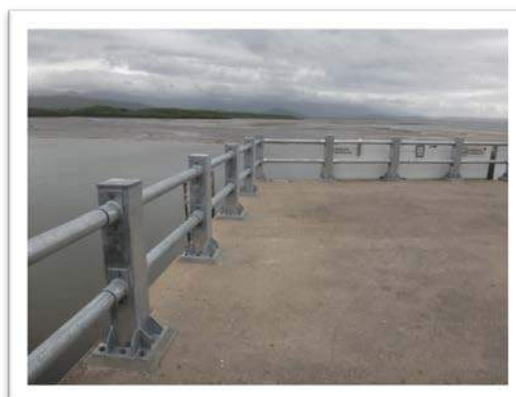
Image: New Vehicle Rails at Sugar wharf
