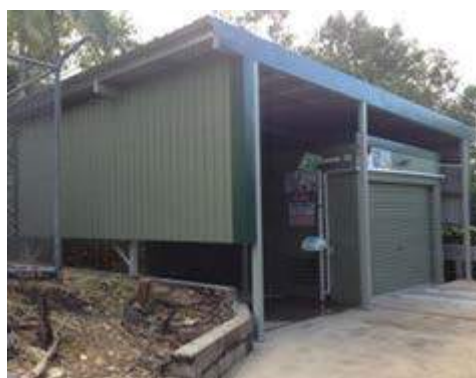
Image: MWTP forklift bay
