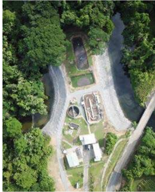
Image: Mossman WWTP Riverbank Stabilisation Project
