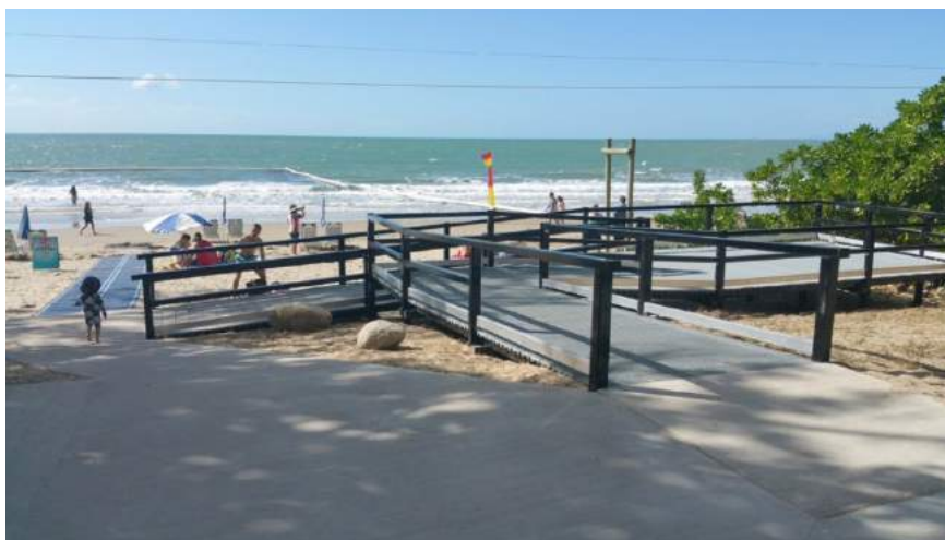
Image: Disability Access Ramp
