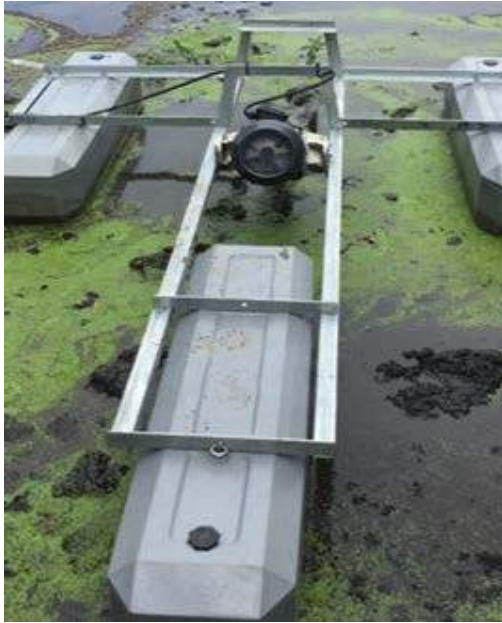
Image: Aerator mixer installed at Mossman WWTP
