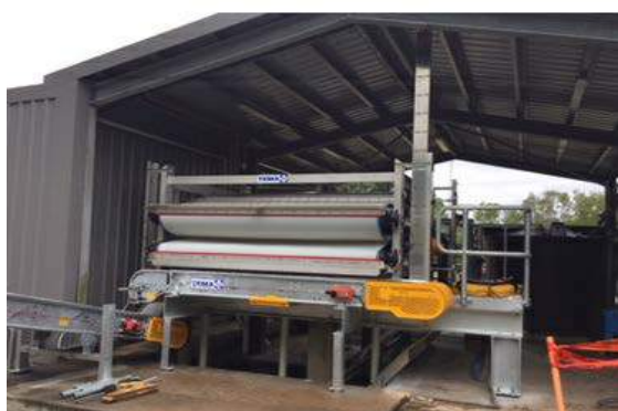
Image: PDWWTP belt press and conveyors installation
