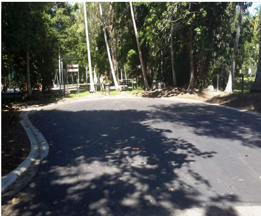
(Above) Solander Boulevard - kerb and channel replacement and asphalt reseal
