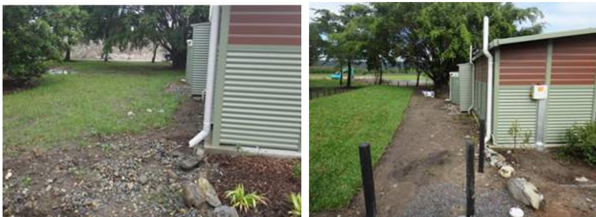
(Above) Gateway Toilet Dispersal area (before and after the project was completed)
