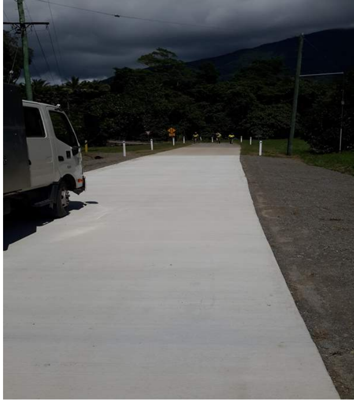
(Above) Kingfisher Lane extension of concrete approaches to bridge
