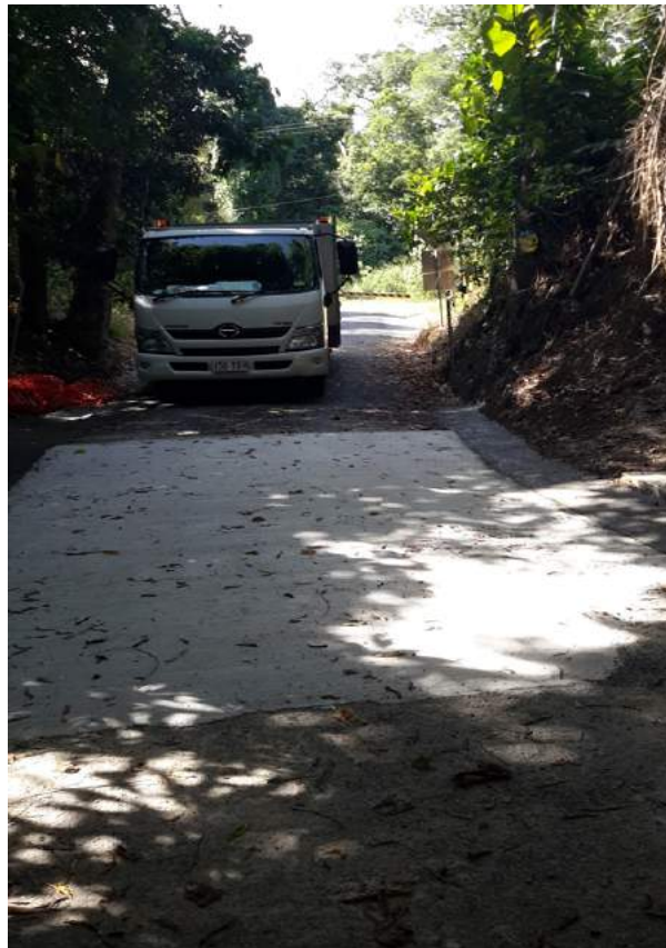
(Above) Old Forestry Road Causeway concrete extension Northern Approach
