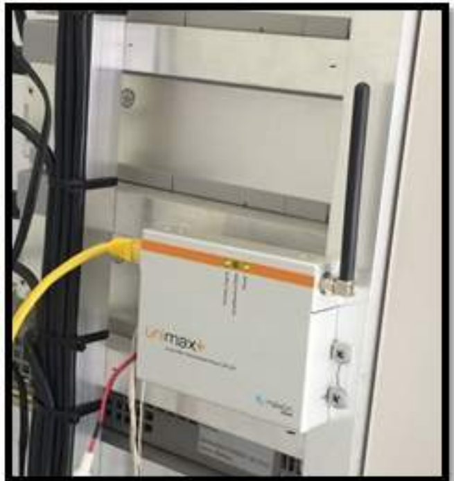
Right: Daintree Modem for remote access
