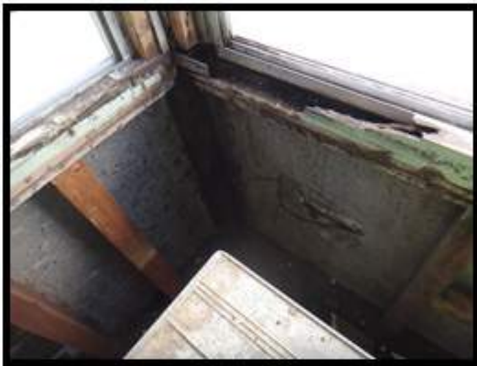
Rotten Timber in Wall
