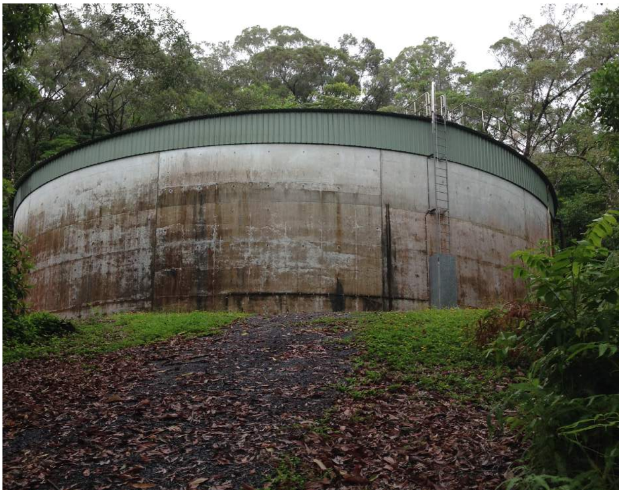
Figure 9 – Whyanbeel Clearwater Reservoir
