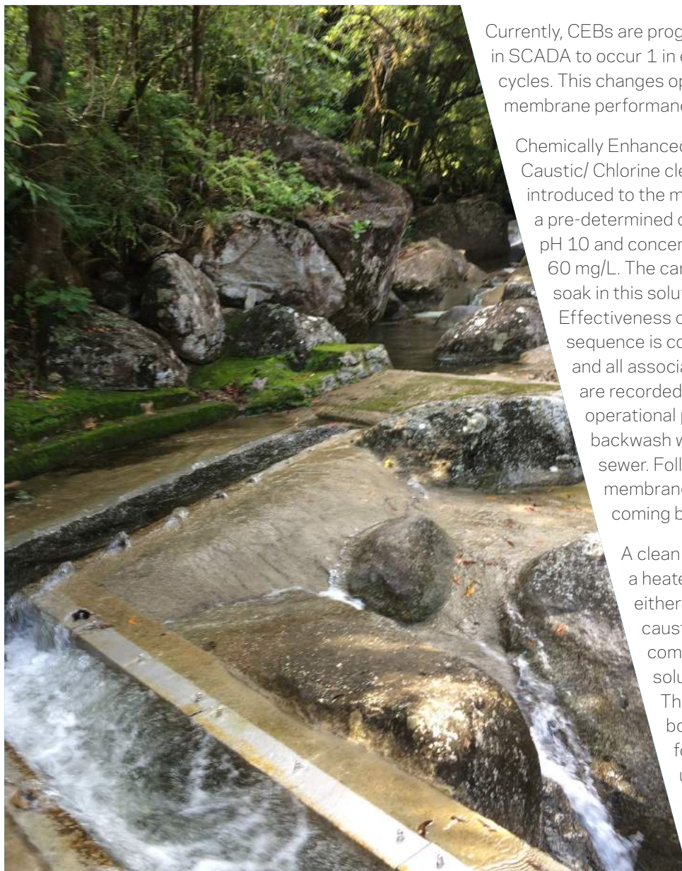
Figure 6 — Rex Creek Intake - race is lined with Stainless Steel
