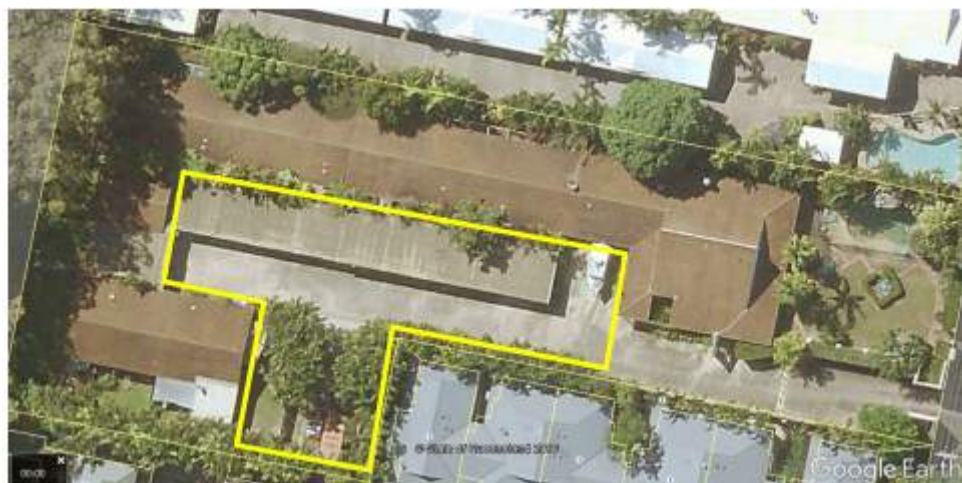
Image 1: Site Aerial (source: Google Earth Queensland Globe December 2016)
