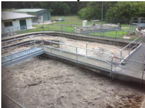
New handrails fitted at Mossman WWTP
