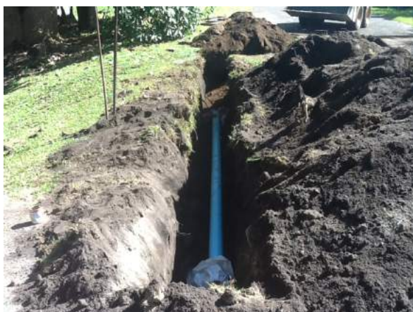
Newell Beach 100mm water main installation
