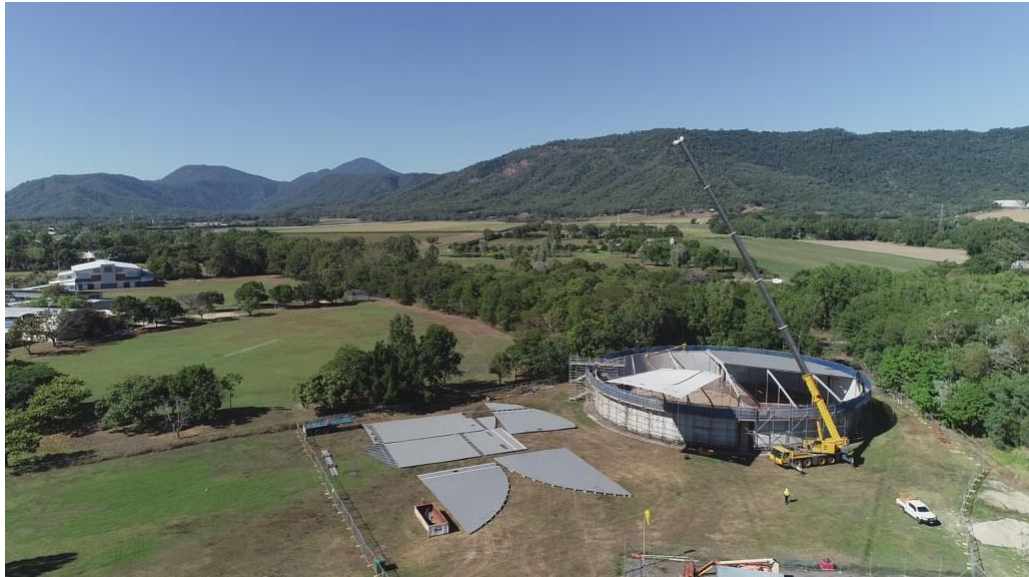
Image: Crane removing large portions of the existing roof
