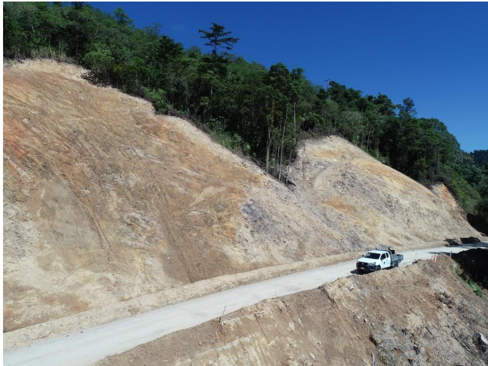
Image: Initial stabilisation and road reopening on Upper Daintree Road
