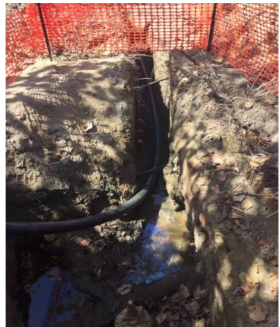
Image: Sewer rising main replacement
