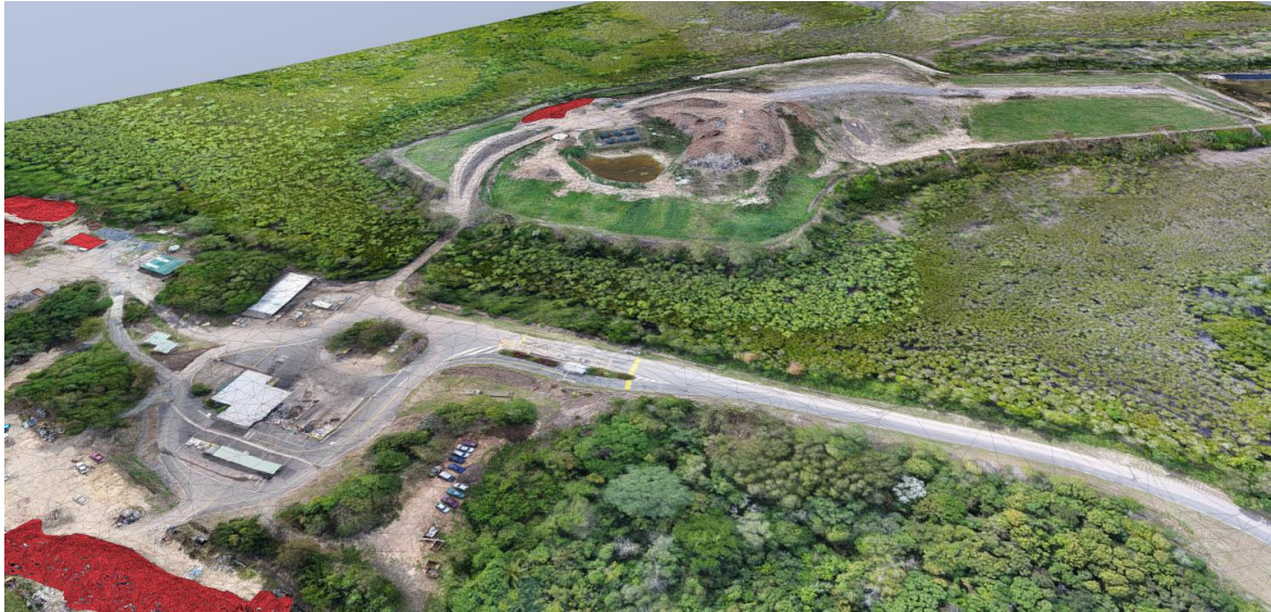
Image: Drone footage from the volumetric survey undertaken at Killaloe Transfer Station & Landfill in August 2019
