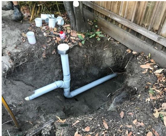
Image 10: Nautilus Street, Port Douglas house connection branch line renewal
