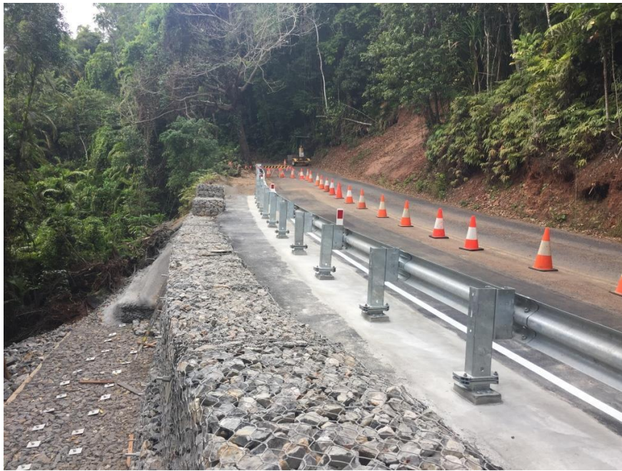
Image: Completed Works
