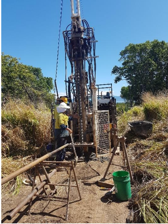
Image: Contractors undertaking Geotechnical work
