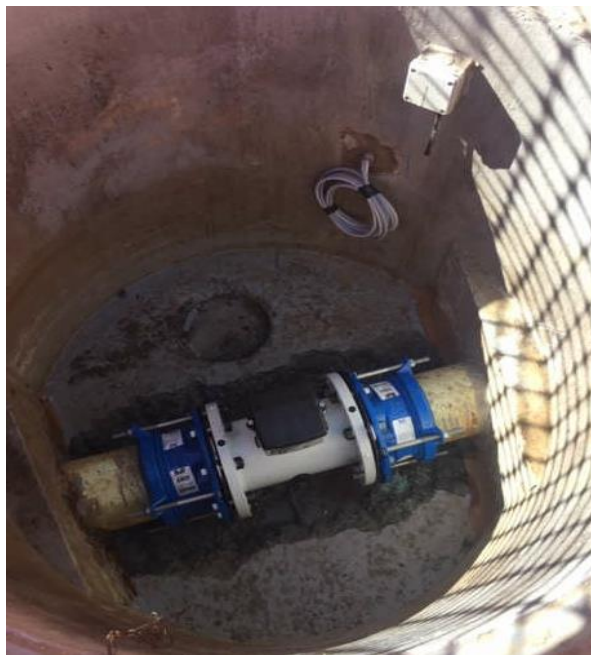
Image: Flow meter installation
