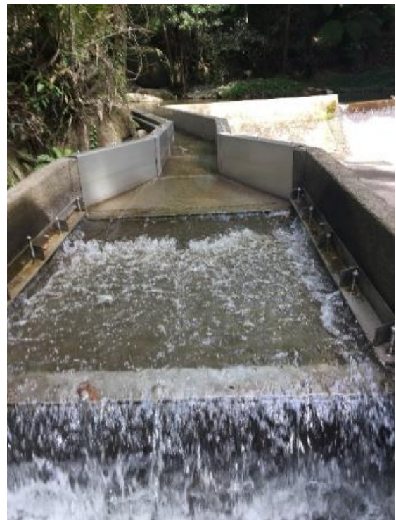
Image: Whyanbeel Creek new screens & race overflow channel
