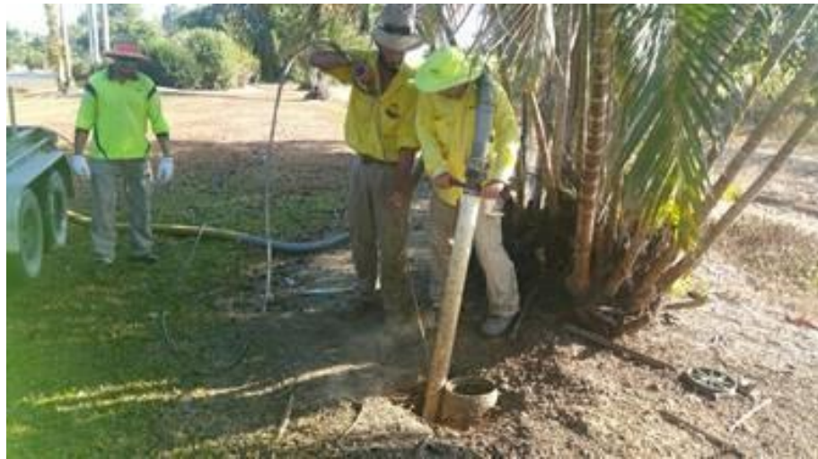
Image: Irrigation repairs
