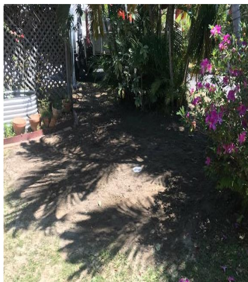
Images: After Port Haven house connection branch line renewal
