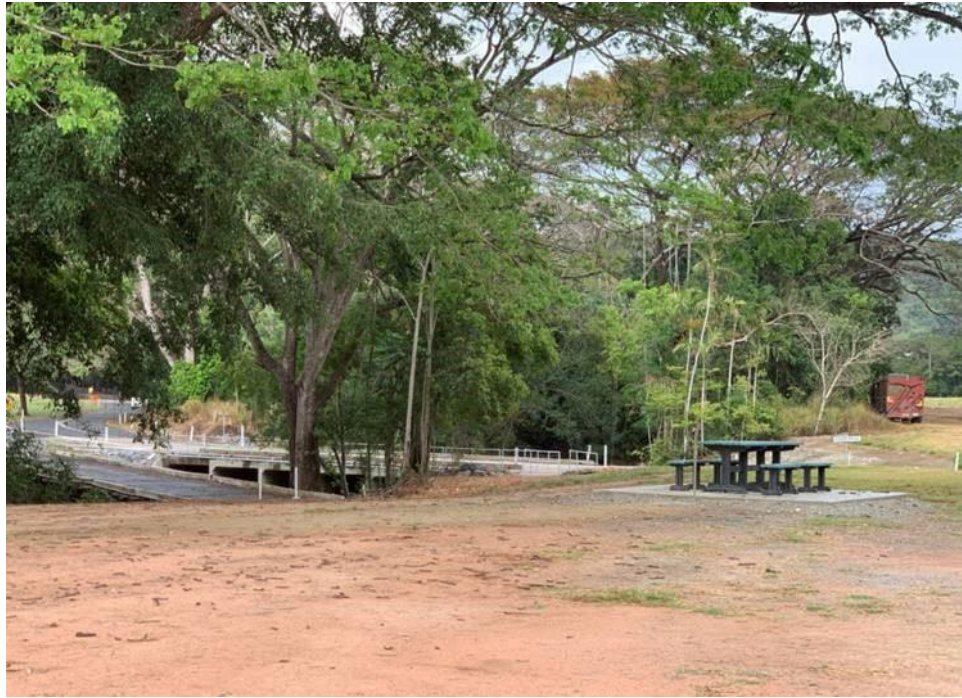
Image: Diggers Bridge pedestrian bridge
