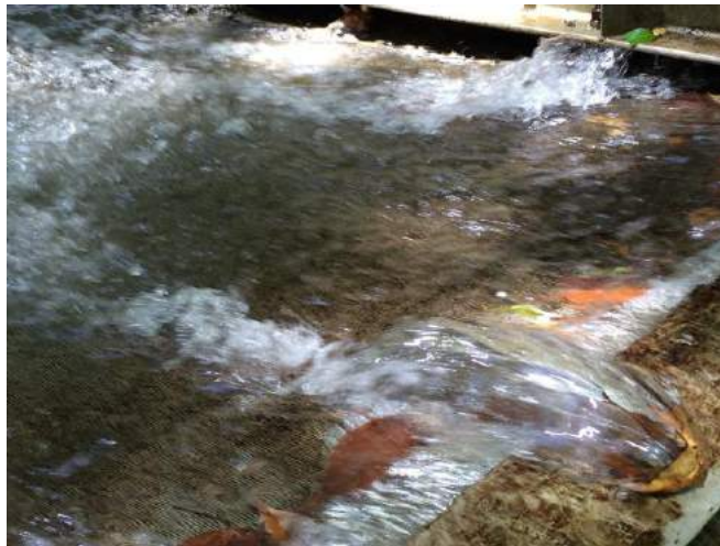
Figure 12 Whyanbeel Intake Johnson Screen
