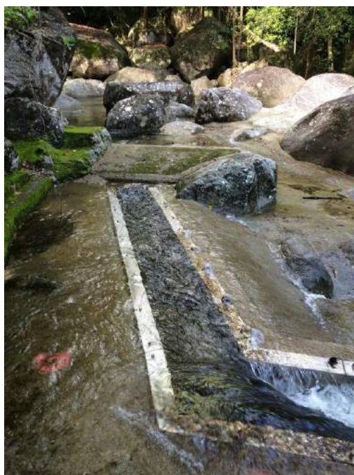
Figure 8 Rex Creek Intake Channel – Mossman
