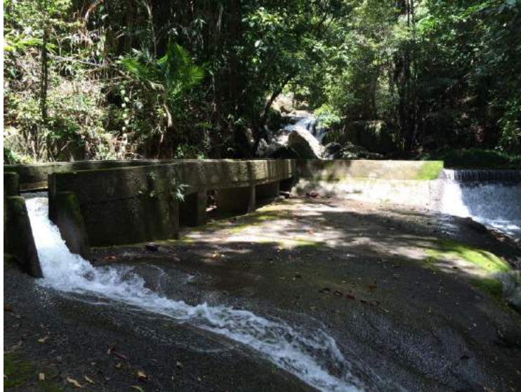
Figure 11 Little Falls Creek Intake - Whyanbeel
