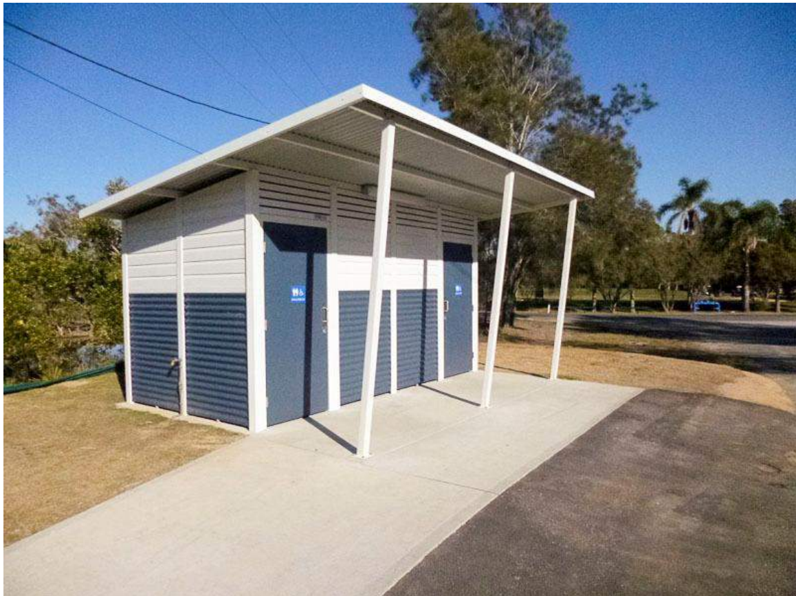
Yarra-2 Toilet Building
