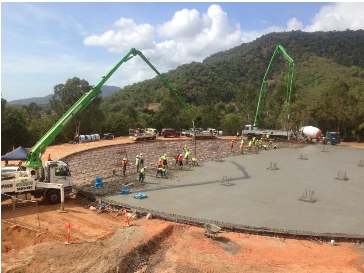
12 September 2017 – Reservoir slab concrete pour
