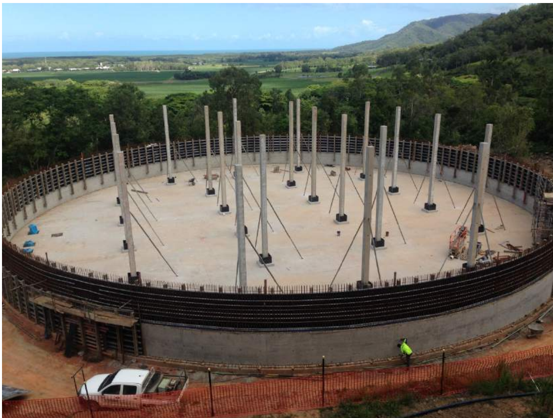
17 November 2017 – Reservoir tank, wall lift #2 underway, internal columns temporarily propped
