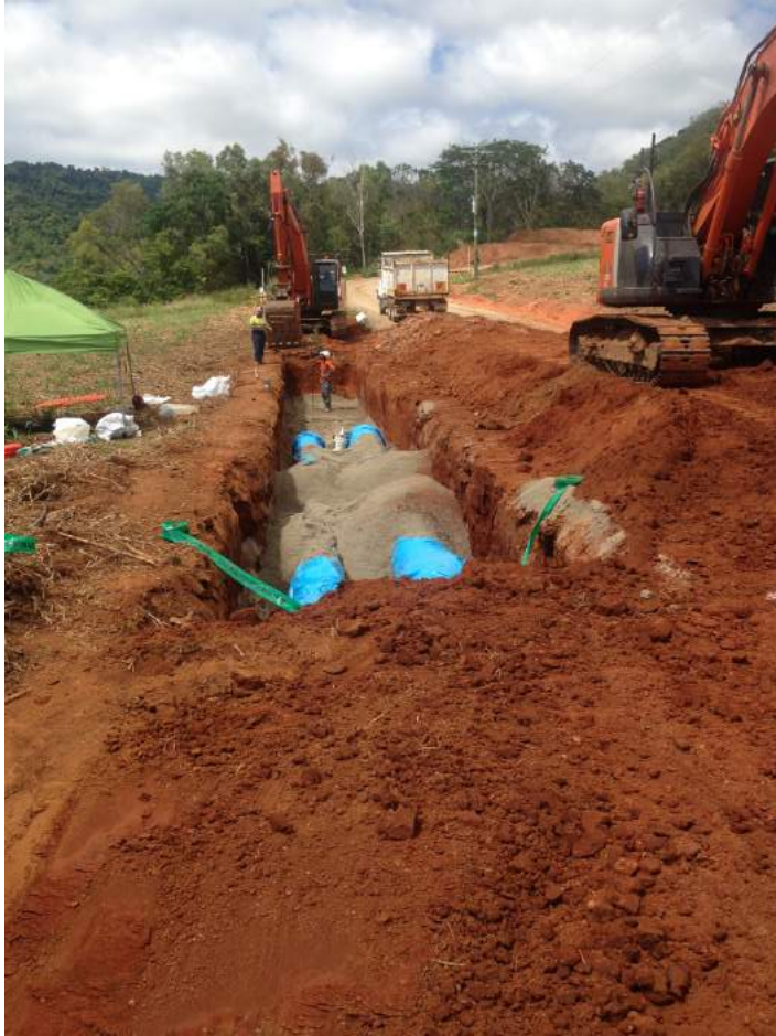
31 October 2017 – 450 and 600mm diameter pipe laying
