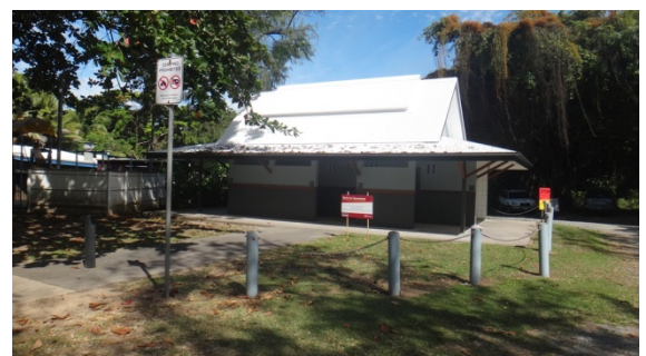
Image: Mowbray St Toilet (Refurbished)
