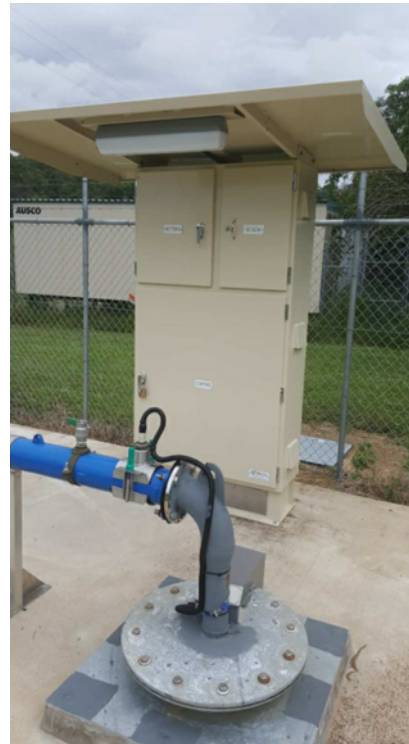
Image 9: Completed Daintree water bore
