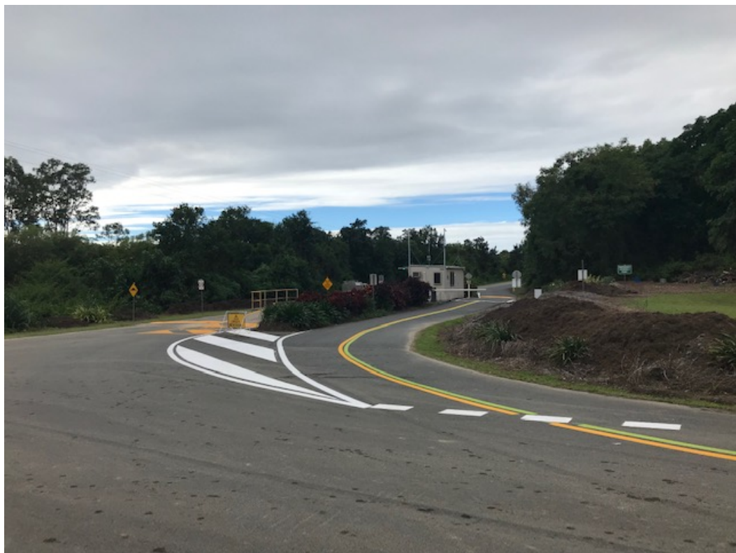
Images: new and refreshed line marking at Killaloe Transfer Station under the LGLRGP.
