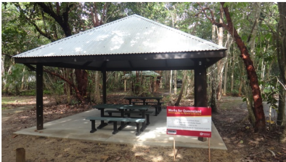
Image: Thornton Beach – New Picnic Shelter
