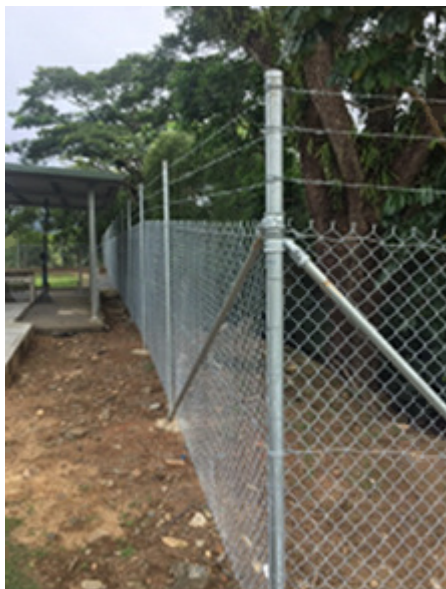
Image 10: Port Douglas WWTP Security Fence
