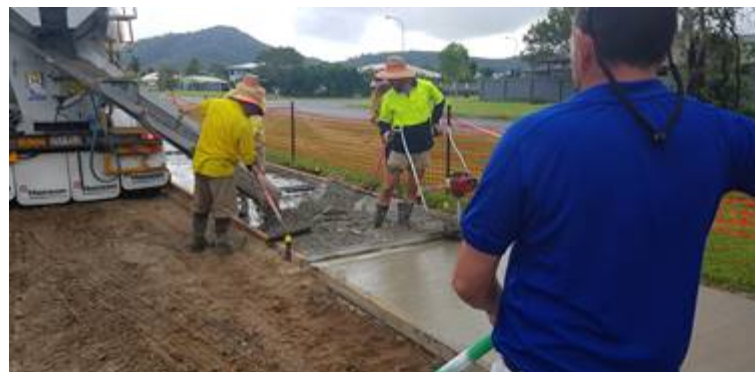
Image: Crews working on the footpath upgrade in front of Mossman Hospital
