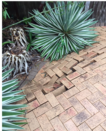
Image 4: Sink hole from a broken house connection branch line
