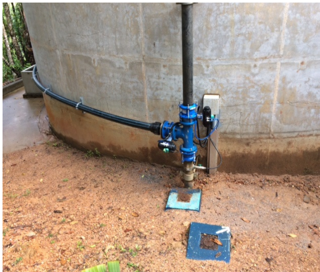
Image 8: Daintree WTP new scour valve
