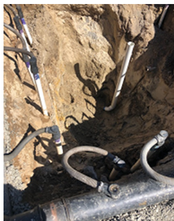
Images 6-7: Andrews Cl, Port Douglas before and after photos – repairing house connection branch lines
