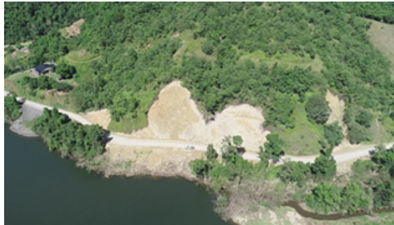
Image: Landslip at Upper Daintree Rd from January 2019 Monsoon event
