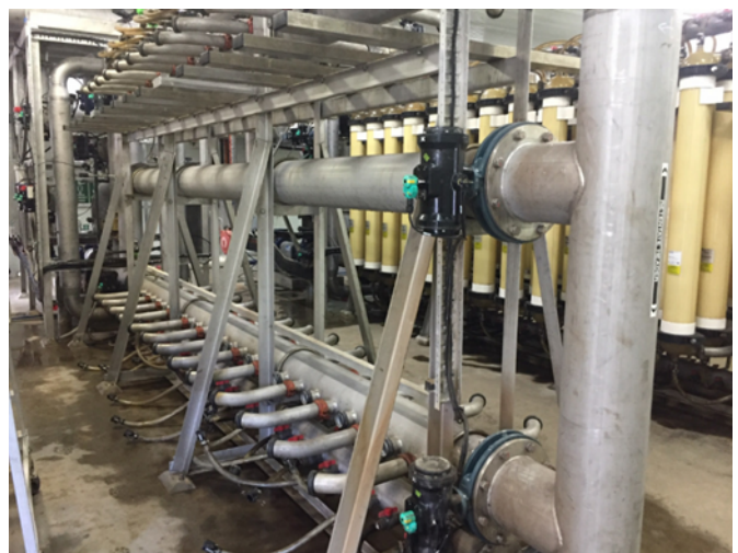
Image 11: Mossman WTP UF cartridges
