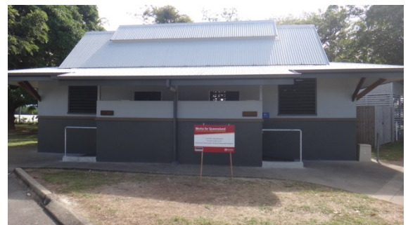
Image: Wharf St Toilet (Refurbished)
