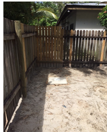
Image 5: Repaired house connection branch line, ground ready to be repaved
