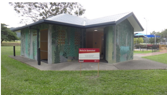
Image: George Davis Park Toilet (Refurbished)
