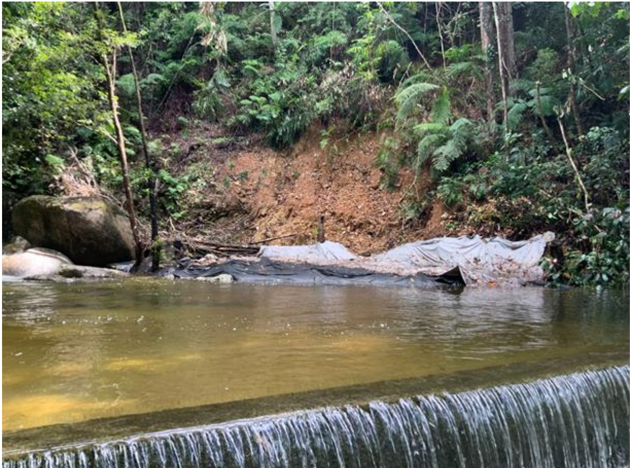
Figure 1. Landslide at Whyanbeel intake
