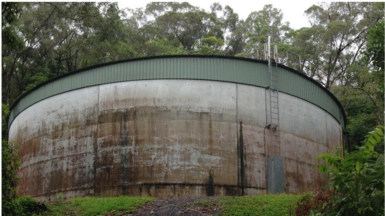
Figure 9. Whyanbeel clearwater reservoir
