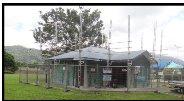
Image: George Davis Park Toilet ready for roof painting.
