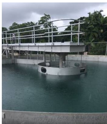
Image: Mossman WWTP new clarifier
