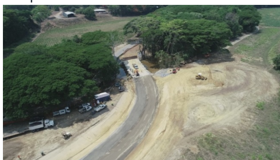
Image: Diggers Bridge Construction Site
