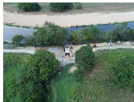
Image: Upper Daintree Culvert Renewal
