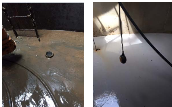
Images: Before and after photos cleaning out of De Meio Reservoir
