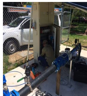
Image: Daintree bore works phase 2
