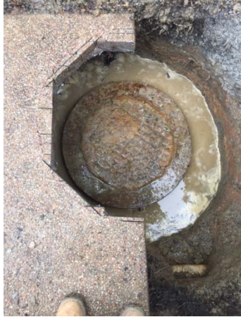
Images: Before and after of a raised manhole in Ulysses Ave, Port Douglas
