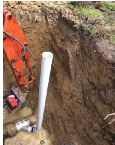
Image: Thomas Street, Mossman house connection branch line repairs
