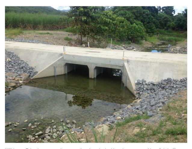
Wilkinson Rd culvert upgrade – completed works looking downstream. Note fish baffles on walls of culvert as per Department of Fisheries requirement
