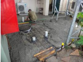
(Above) Concrete removed ready for new grease trap & new concrete being installed.
