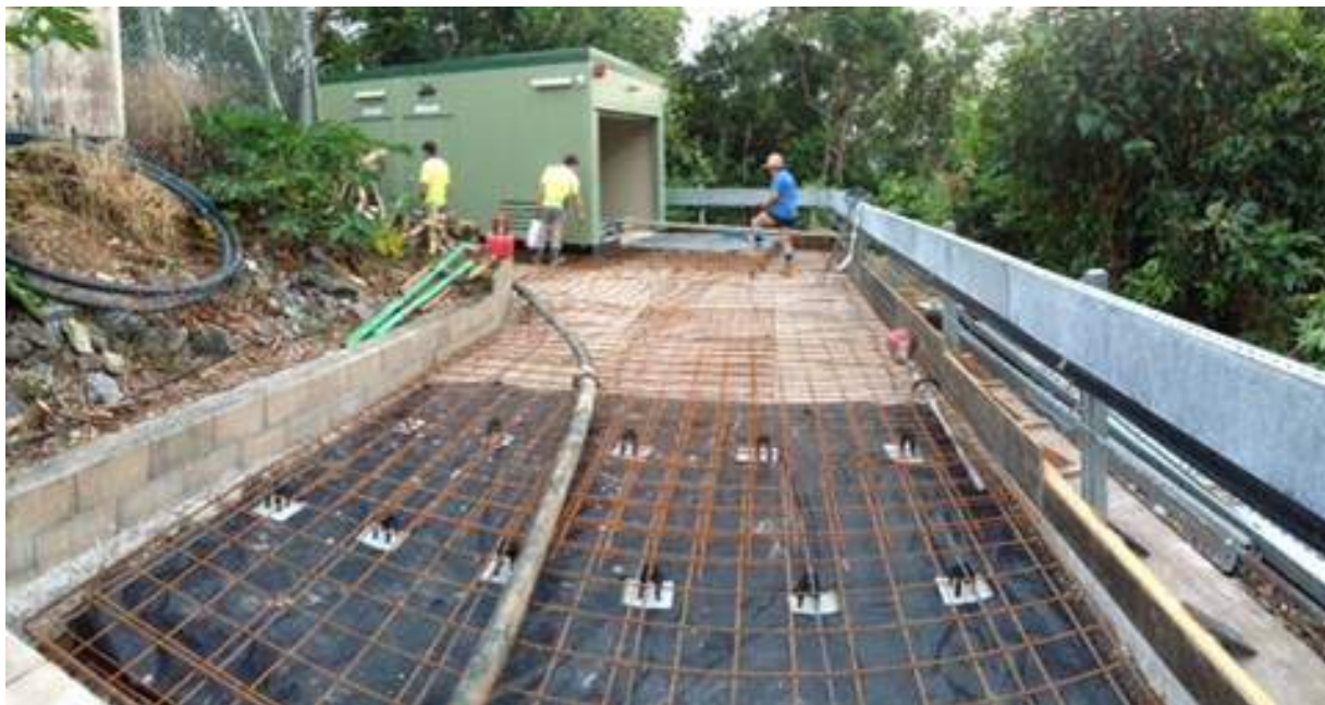
Image - Mossman WTP Concrete Slab Pour – Gas Chlorination Plant Installation
