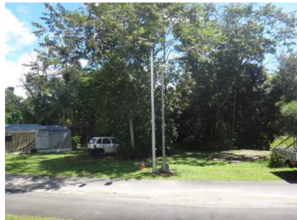
New Light pole beside old before its removed.
