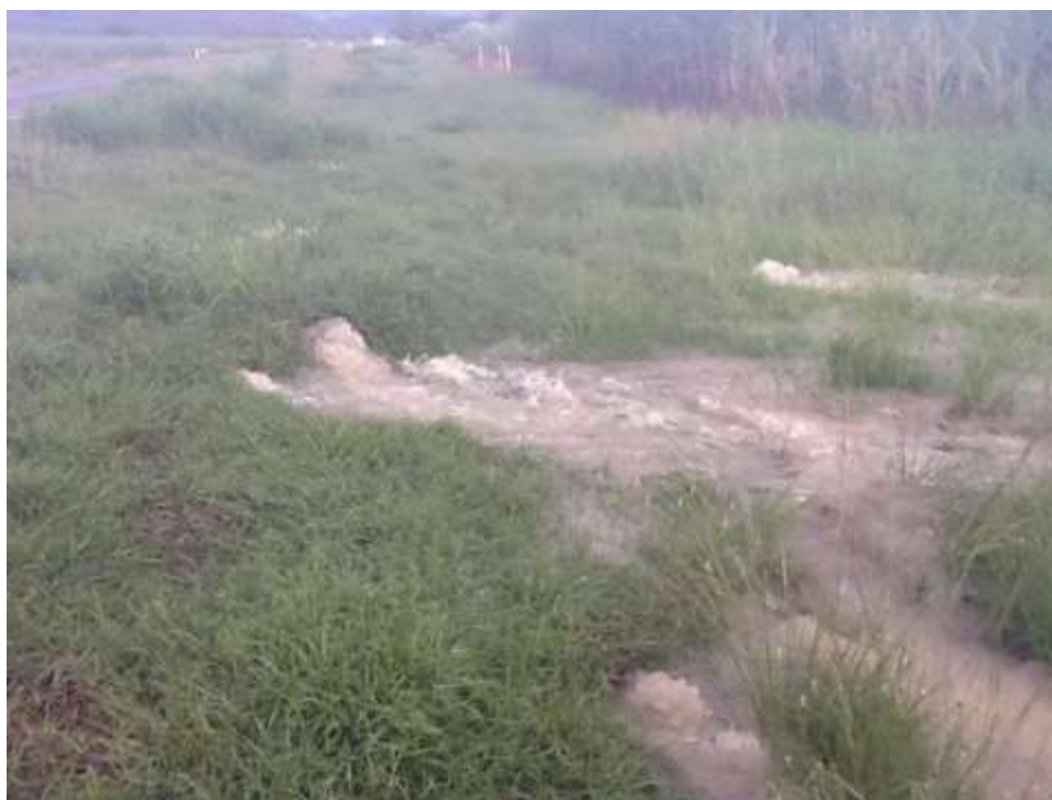
(Above) Example of break in water main
