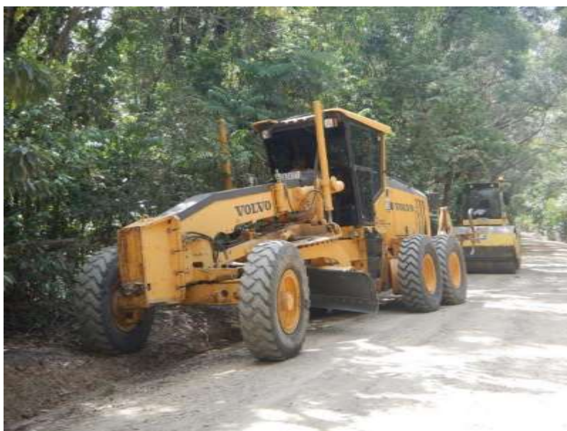
(Above) Road grading crew completing the gravel re-sheet program north of the Daintree River
