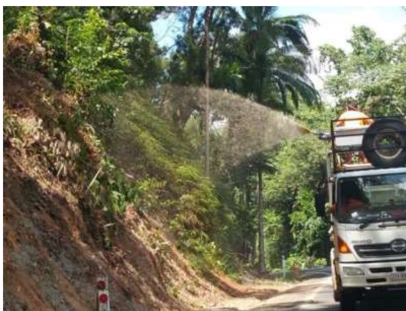
(Above) Hydro mulching of bank stabilisation project for DTMR at Humbug Reach
