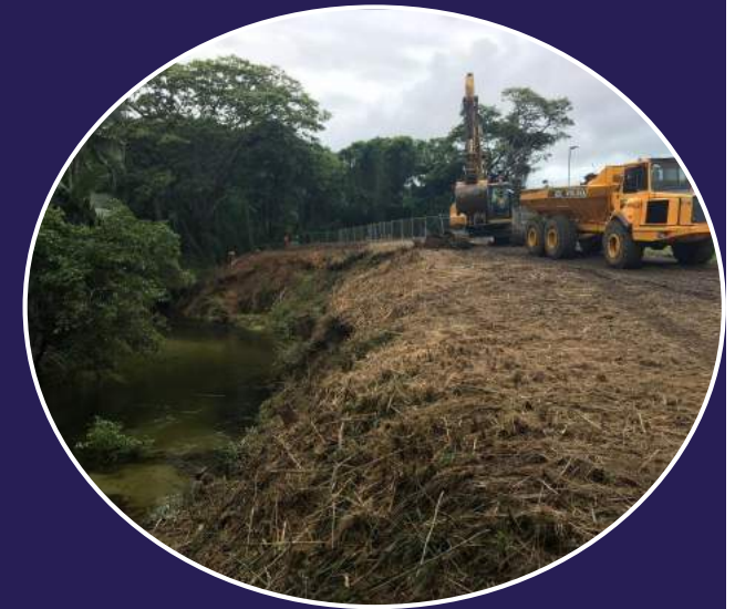
River bank stabilisation conducted near Mossman wastewater treatment plant
