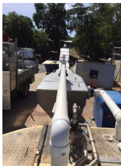
Image: Port Douglas wastewater treatment plant grit classifier installation
