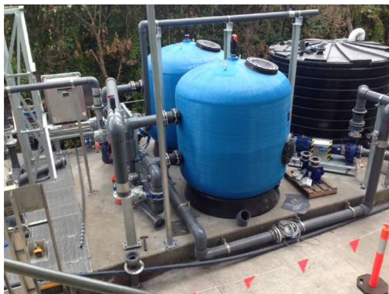
Image: Mossman water treatment backwash water discharge reuse package plant
