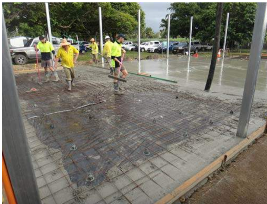
Image: Council Concrete crew pour the new depot lunchroom floor.
