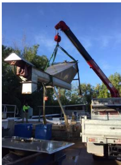
Image: Port Douglas wastewater treatment plant grit classifier installation
