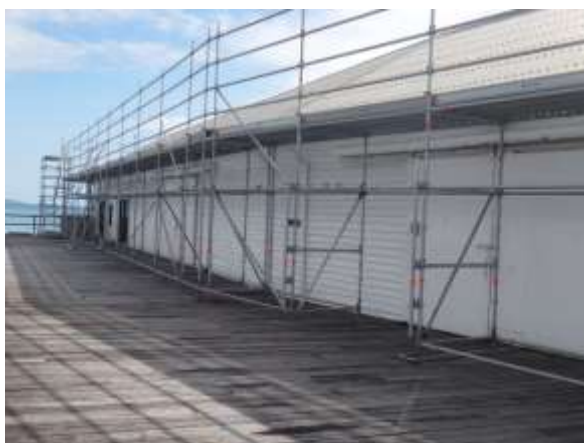
Images 50 and 51 (above) Scaffolding for Port Douglas Sugar Wharf Roof replacement
