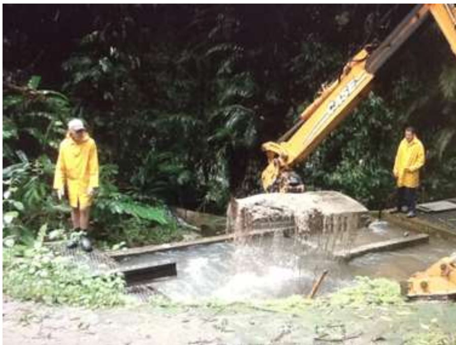
Image 54 - (above) Intake clean up during wet weather event
