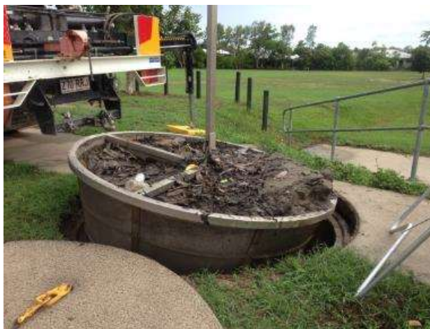
Image 30 – (above) Gross Pollutant Trap being cleaned
