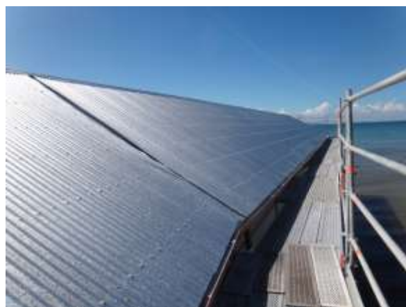
Images 52 and 53 - (above) New Heritage Z600 Galvanized iron fitted to the Port Douglas Sugar Wharf Roof
