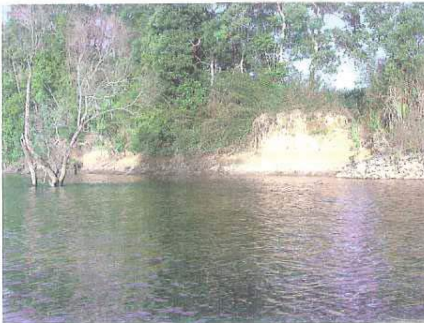
Another view of the severe erosion that has now developed where the rockwork was not completed in 2004.
