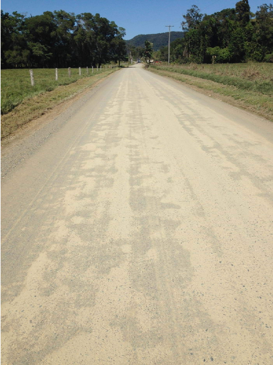
Forest Creek Rd Ch 5.110-Ch5.710 – Completed gravel resheet
