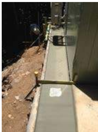
Mossman WTP Slab for New Forklift Bay
