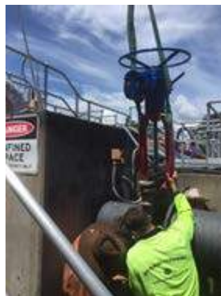
SBR Inlet Valve Installation
