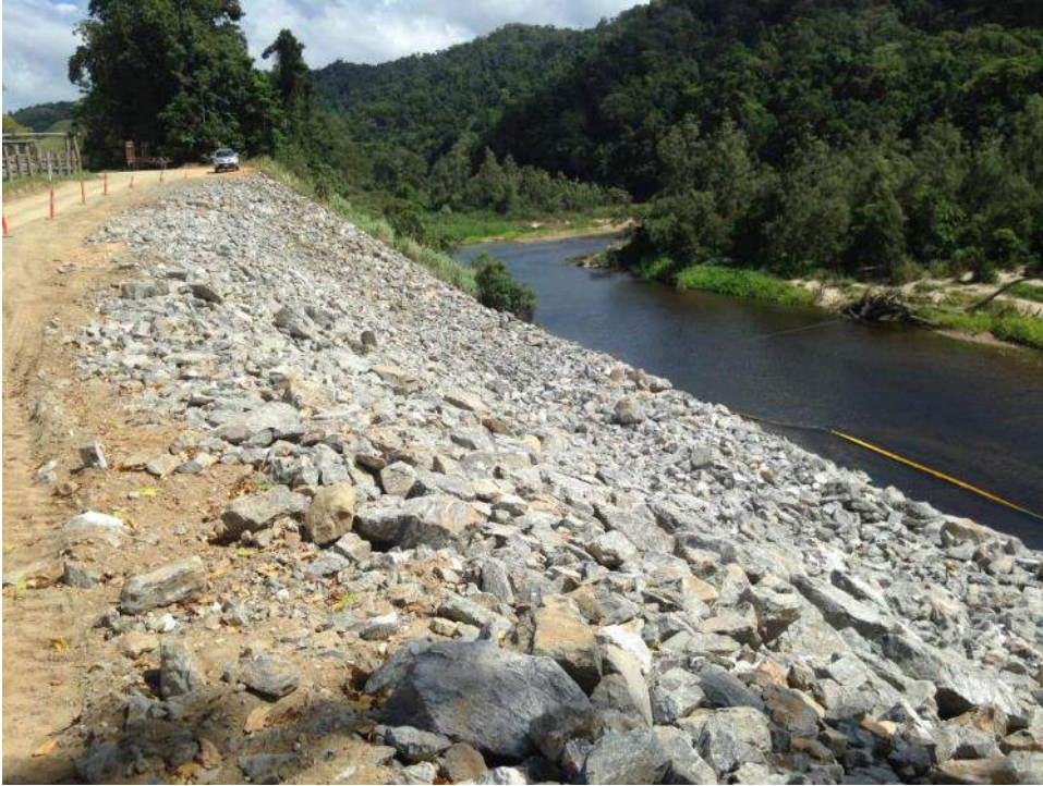
(Above) Landslip stabilisation - Upper Daintree Road adjacent to Daintree River
