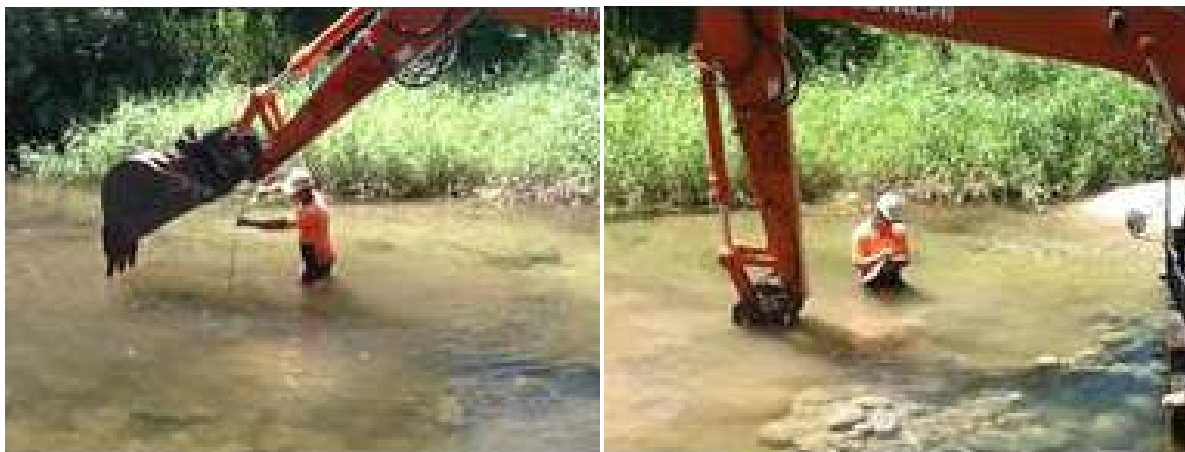
(Above) Preliminary geotechnical investigations in the Mossman River as part of the water security project
