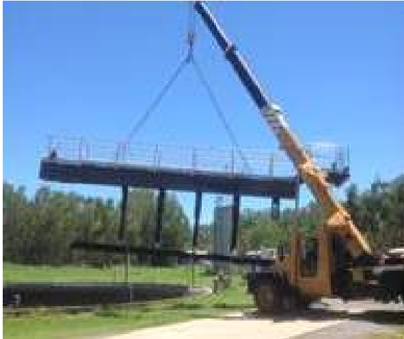
(Above) Equalisation bridge removal
