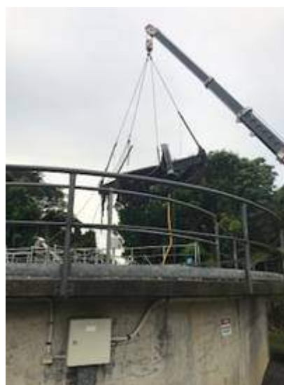
Image - Mossman WWTP Diffuser Replacement
