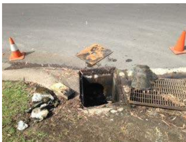
Image - Steel plate, lumps of concrete and timber was just some of the items removed from the drain.
