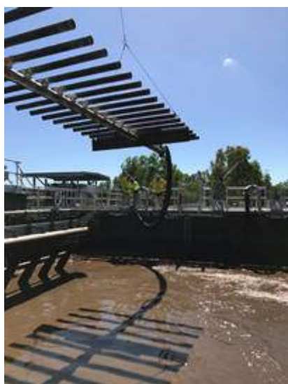
Image - Port Douglas WWTP Diffuser Replacement
