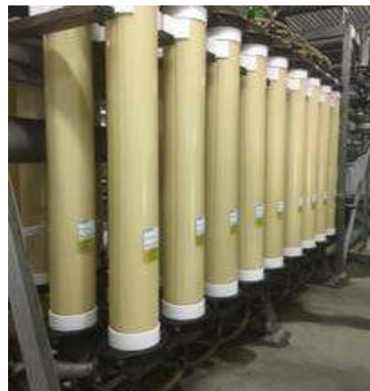
Image - Whyanbeel WTP UF Cartridges Replacement
