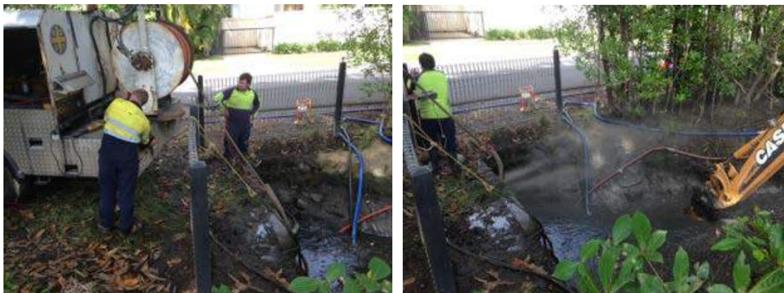
Images - Backhoe assisting in removing the large amount of sand and other debris
