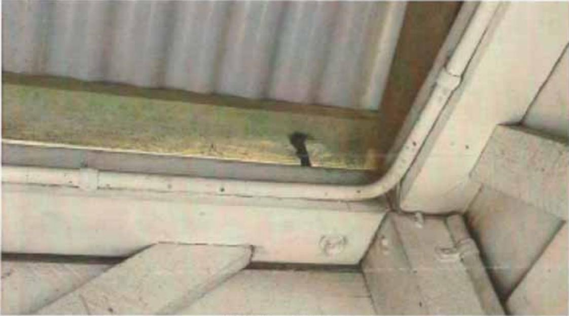
Corroded roof fixings
