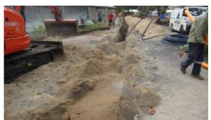
(Above) New Power Conduit being run between the two Toilet Blocks
