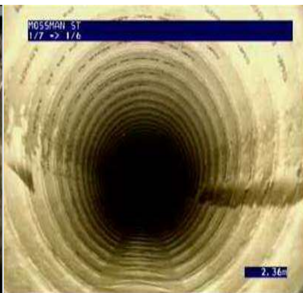
(Above) Sewer pipeline after relining
