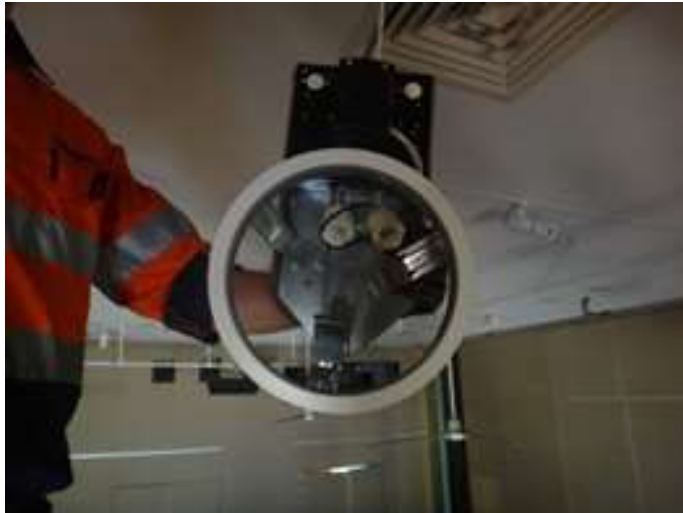
(Above) Old Twin Fluro Type Down light being replaced
